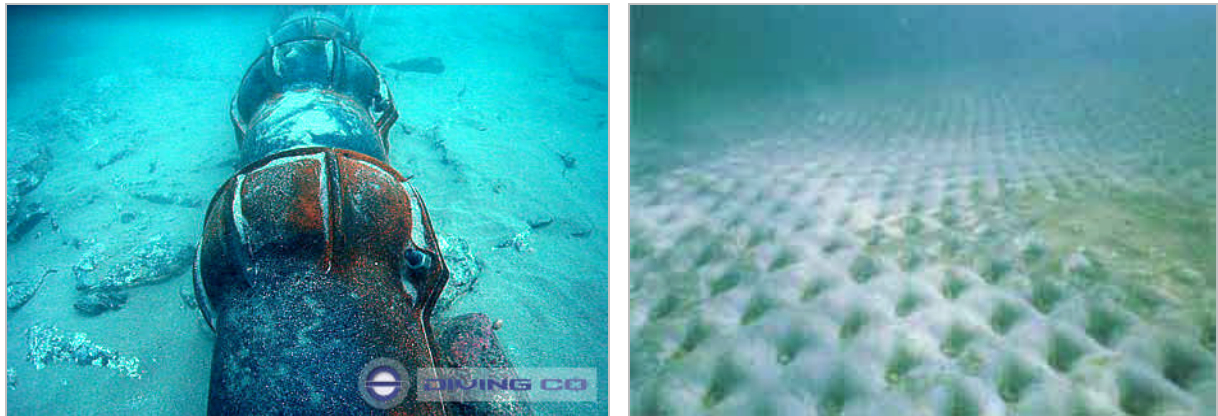
Fig. 13 Left: Basslink cast iron shell cable protection ( www.divingco.com.au ), Right: Flexitex concrete mattresses for cable protection ( http://www.marinetrench.com/alternative.html ).
