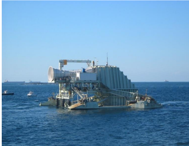
Figure 5: A Wave Power Station in South Australia [8]
