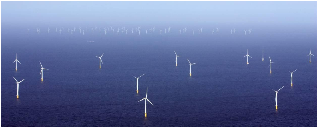
Figure 54. Aerial view of OWEZ in the foreground and PAWP in the background. Photo Hans Verdaat, IMARES, 7 July 2010.
