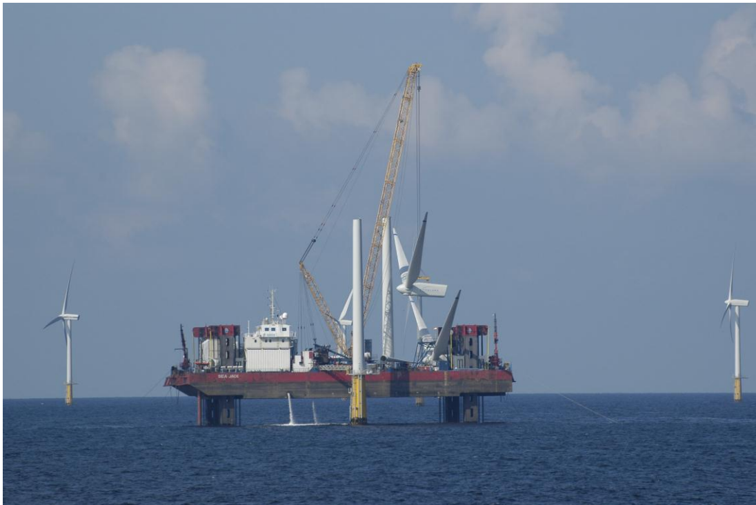
Figure 6. Construction activities in PAWP: preparations for hoisting a turbine. Building PAWP took place while OWEZ was already fully operational and while T-1 seabirds surveys (see main text) for OWEZ were conducted. Photos: Hans Verdaat, IMARES (top) Kees Camphuysen, NIOZ (bottom).
