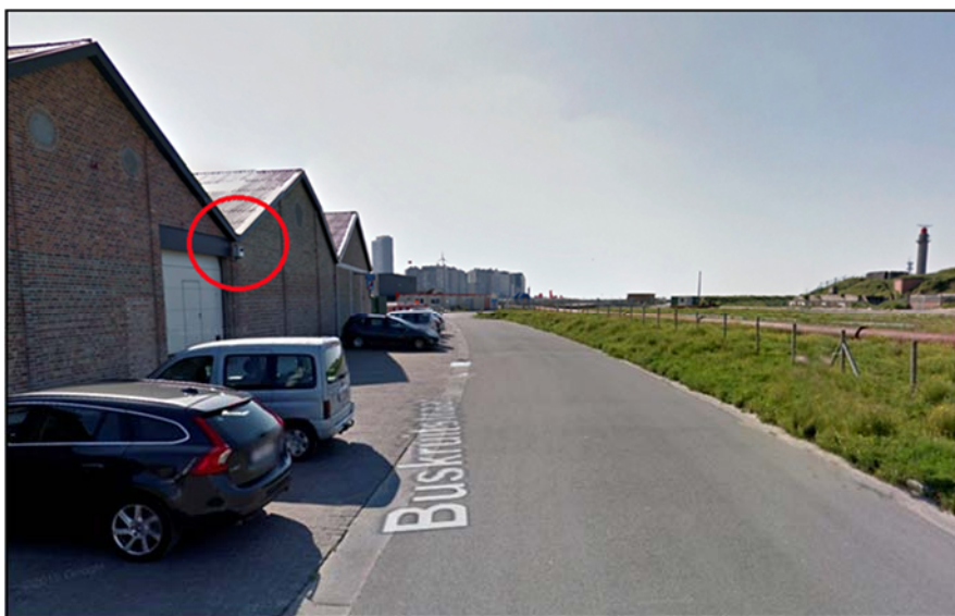
Figure Annex 1-10. Monitoring location Oostende in 2015 (photo: INBO).
