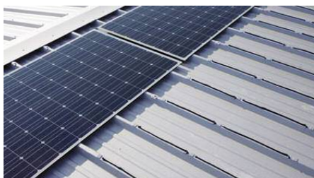
Figure 2.2 The SOLBOND system PV panels bonded to a standing seam metal cladding roof system.
