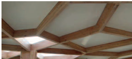
Figure 2.13 Glulam beams in the Sumika Pavilion.
