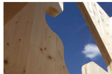
Figure 2.16 CLT construction of the MK40 tower.
