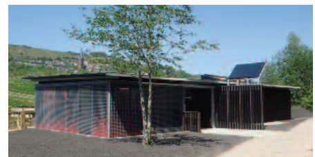
Figure 2.20 Ty Unnos Ebbw Vale Classroom.
