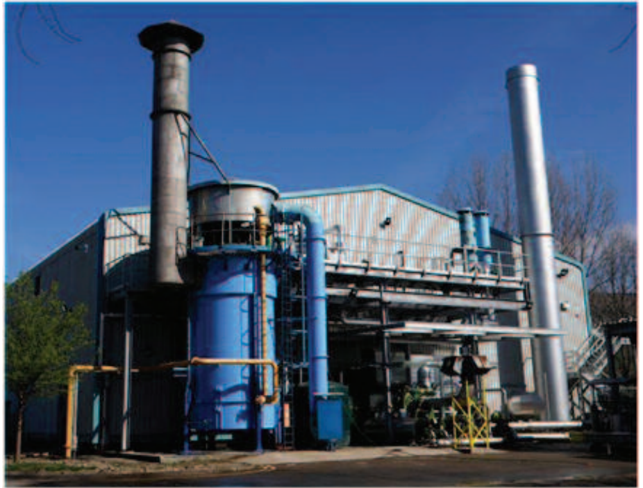
Figure 5.1 The Gas Turbine Research Centre at Margam.
