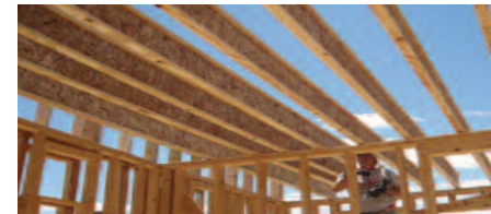
Figure 2.14 Lightweight I-Joists installed in place of traditional solid timber joists.
