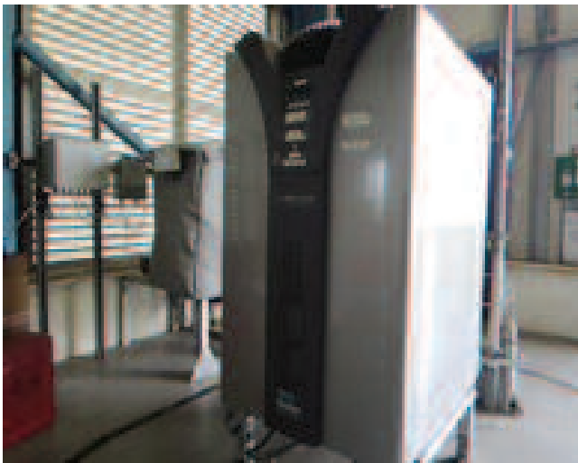
Figure 4.16 SERC developed a building scale hydrogen energy storage test rig, with ITM Power.
