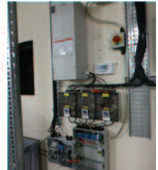
Figure 3.5 Schematic of the DC lighting circuit with supply from the OptIC PV wall and battery storage with picture of the DC battery charger taking the power from the OptIC PV wall.
