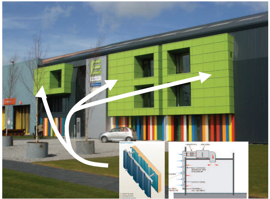
Figure 2.22 SBEC building with its TSC thermal air collectors forming the façade..
