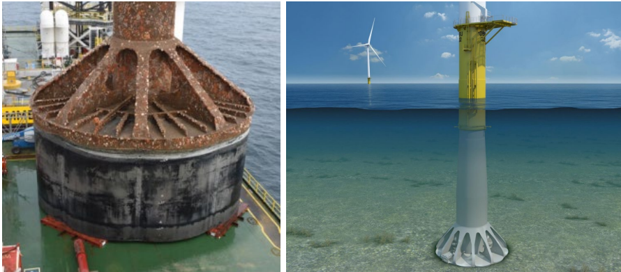
Fig. 14. Installation of a Mono Bucket after full decommissioning (left). Design of a Mono Bucket carrying a wind turbine (right) , ©Universal Foundation.
