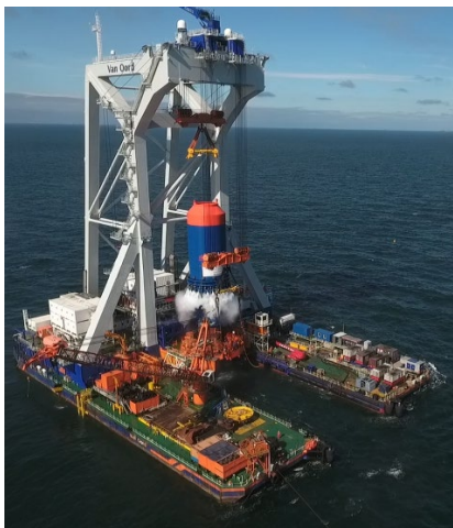
Fig. 9. Draining of seawater from BLUE 25M hammer upon completion of piling operation (left). Frequency spectrum of BLUE piling compared to impact piling at two reference piles (right, note different dimensions: BLUE Piling test: \varnothing 6.5 m, water depth 22 m; reference Gemini OWF: \varnothing 6.6 m, water depth 30 m; reference Q7 OWF: \varnothing 4 m, water depth 19-24 m), © Fistuca BV.
