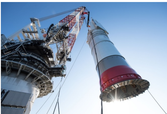
Fig. 3. Monopile installation at the OWF Borkum Riffgrund 1 using the Integrated Monopile Installer with NMS (left, © Ørsted). Frequency spectra (SEL third-octave band level) of ramming noise with and without NMS at OWF Borkum Riffgrund 1, measured 750 m from the pile given as percentiles (right, Gündert et al. 2015).
