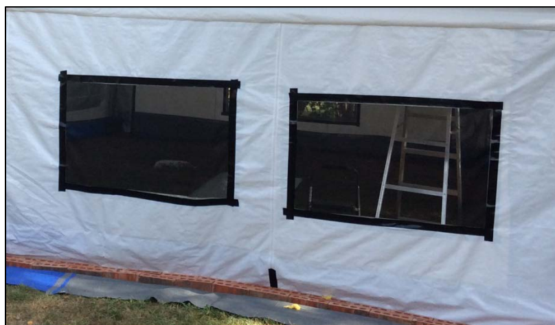
Fig. 3. Mesh covered windows allow natural ambient conditions within the flight facility.
