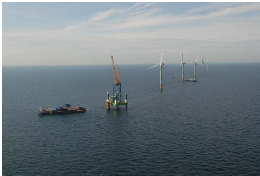
Figure 3. Image of the activity at the Thorntonbank windfarm site on 9 September 2008, showing the cable barge which was also present on 10 September, when underwater noise measurements were made (photo MUMM / RBINS).
