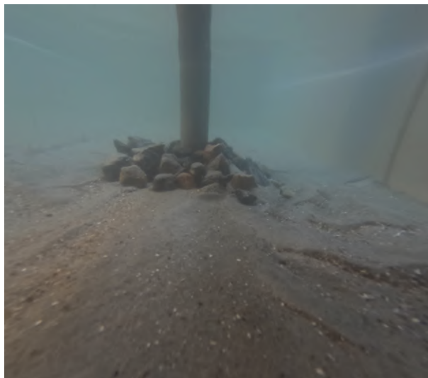
Figure 4.22: View of the surroundings of the tower from the back.
