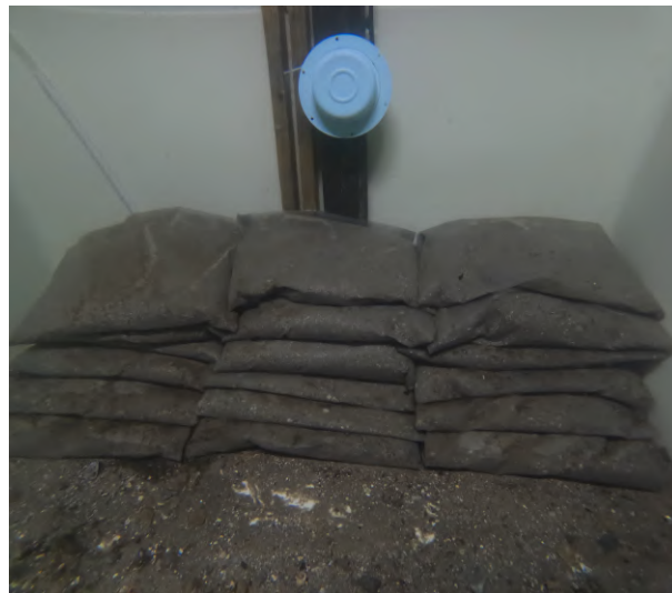
Figure 3.2: Picture of the GTSC scour protection. The underwater speaker can be seen above the scour protection.
