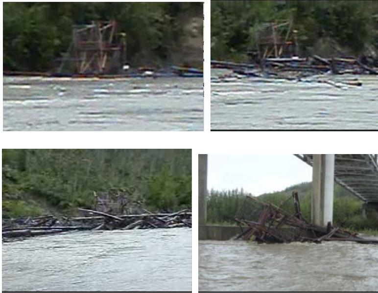
Figure 17. Log debris island impacting (upper left ) and carrying off (upper right and lower left) a fish wheel on the Tanana River near Nanana, Alaska, on August 1, 2008, and depositing it against a bridge pier (lower right) (courtesy of Stephen Lord)
