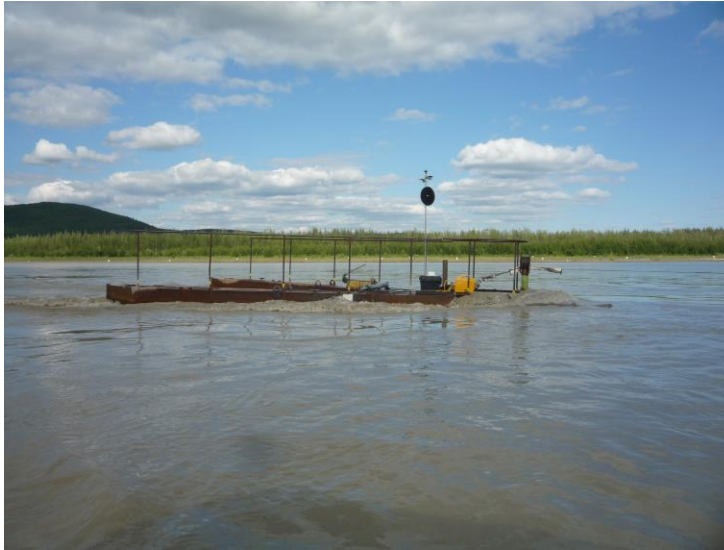
Figure 2. RDDP with nose pitched forward due to high river velocity prior to installation of ballast plates.
