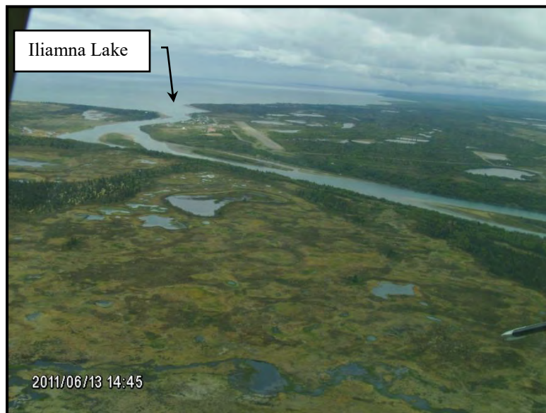
Figure 2 – Aerial view of the project site from the west.
