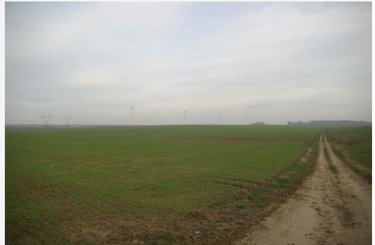
Portes de Champagne wind power project after the application of mitigation Source: ©EDF EN.
