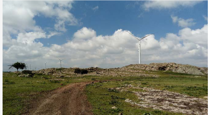
View of the Kipeto wind farm site, central Kenya Source: © David Wilson
