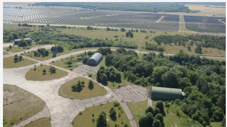
Photovoltaic power plant has given a second life to a former military base in disuse along with pollution abatement of the field
