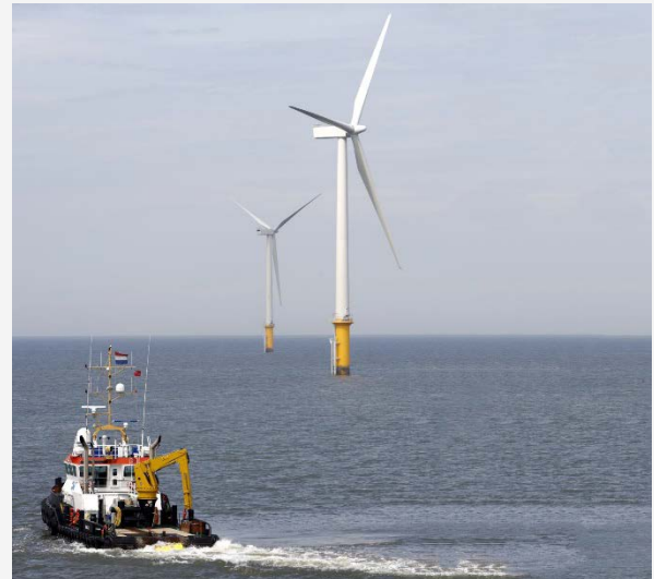
Offshore wind turbines in North Sea Photo: © WindEurope
