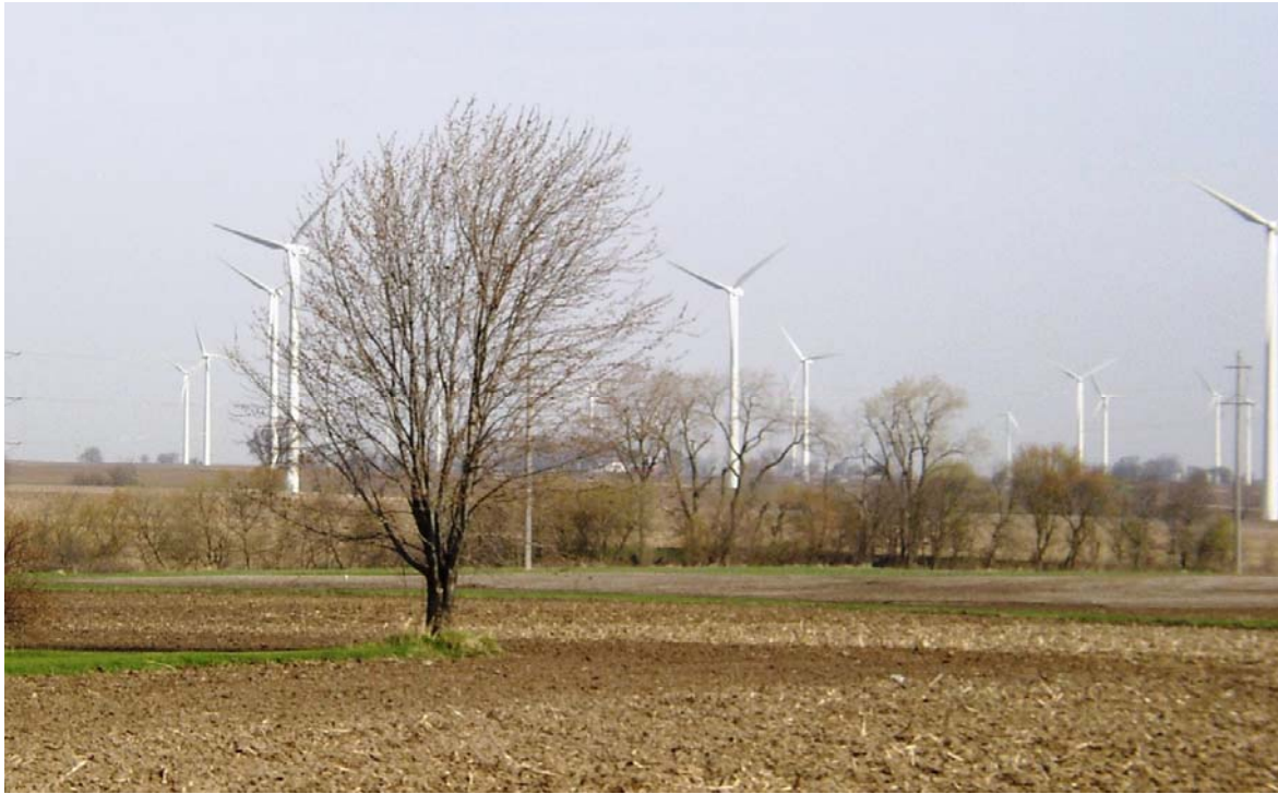
Figure 8. The 800 kW turbines at Mendota Hills are the smallest size generally used in a utility-scale project. Photo: Penny L. Shank
