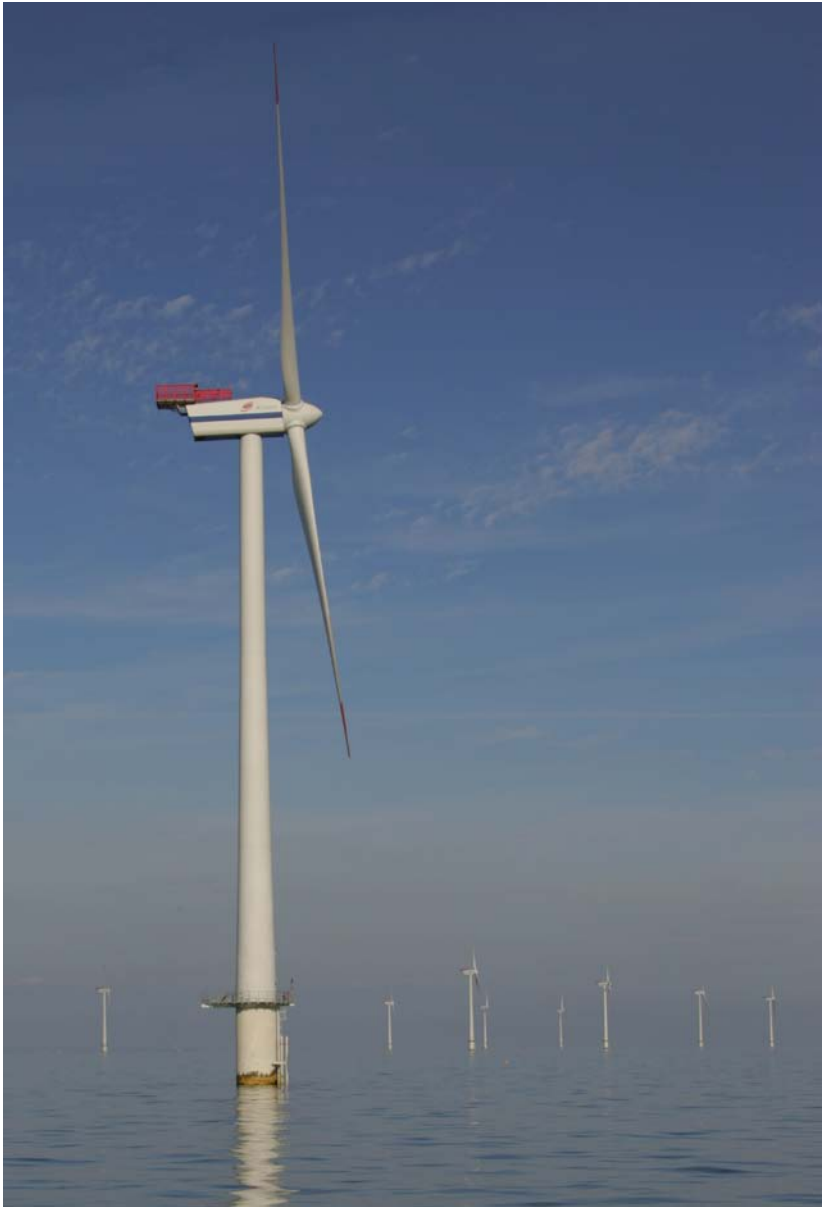
Horns Rev I Vestas turbine
