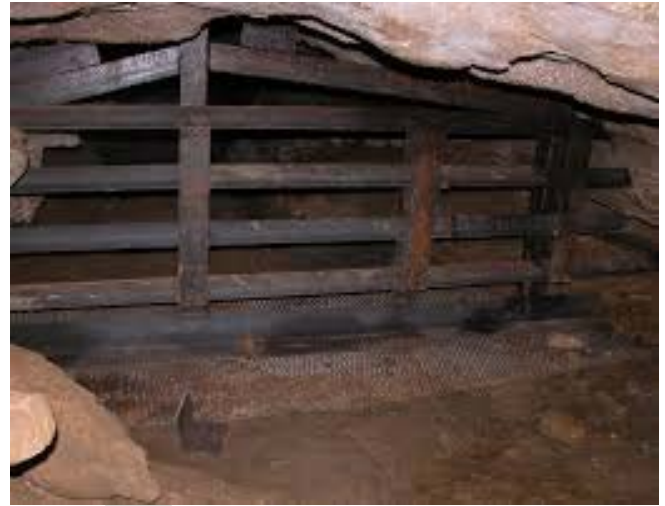
Bat friendly gate installed at cave entrance to deter disturbance of hibernating bats. Photos by Steve Widowski.
