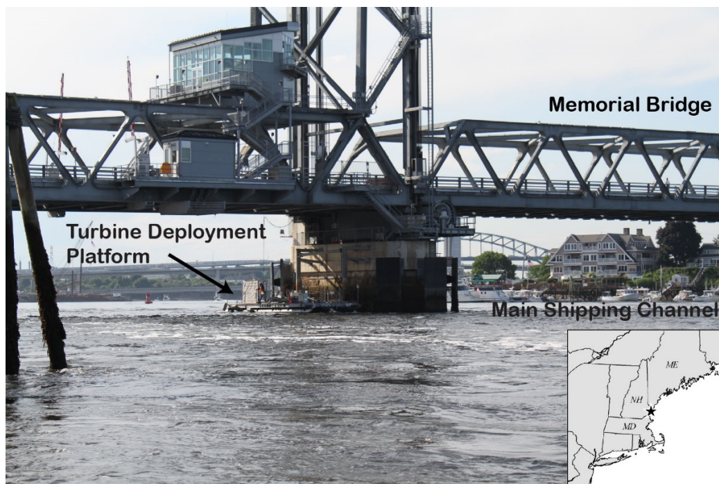
Figure 1. The University of New Hampshire’s Living Bridge Project turbine deployment platform is moored to a pier of the Memorial Bridge that spans the Piscataqua River and tidal estuary on the border of New Hampshire and Maine in the northeastern United States. The star in the lower right inset map represents regional reference location of the site.
