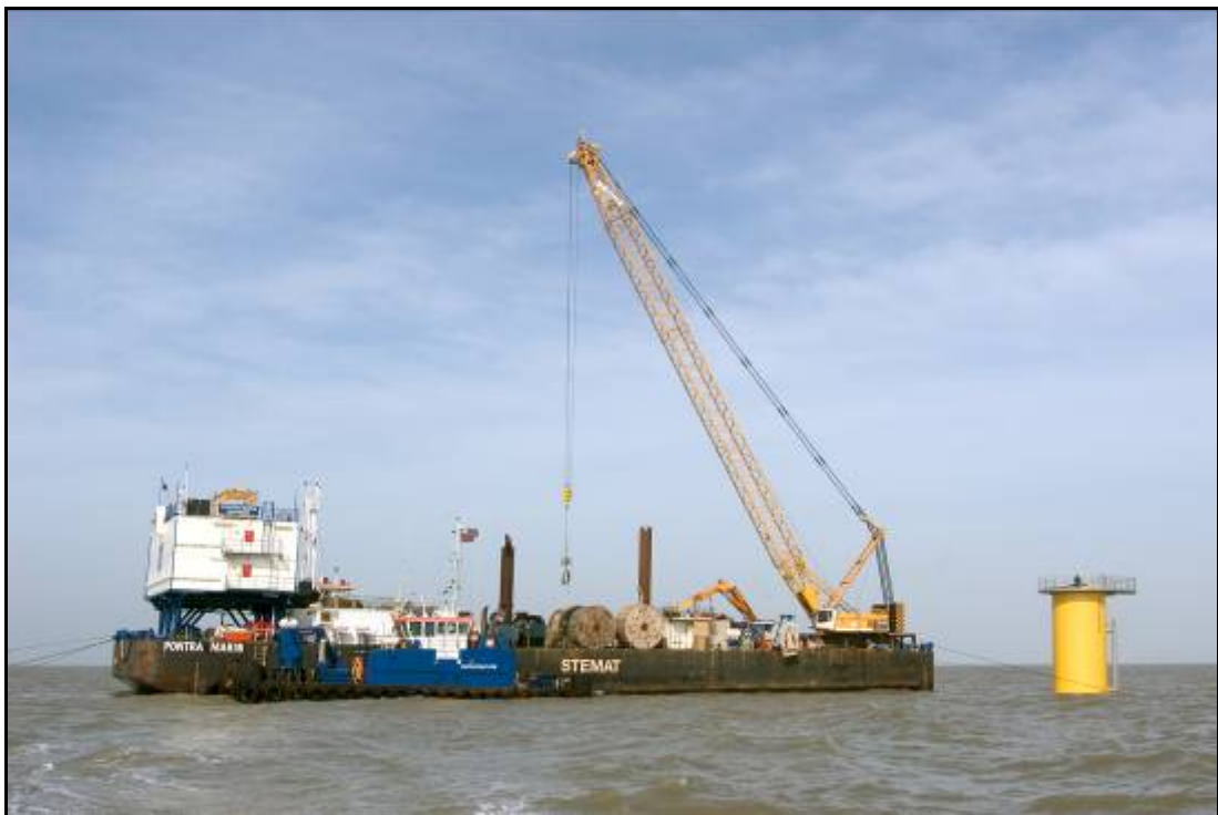
Plate 2.5 Cable laying barge, engaged in cable installation operations at Kentish Flats
