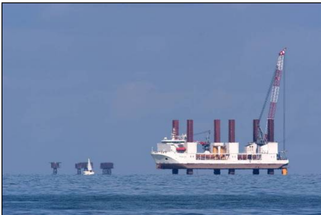
Plate 2.2 Jack-up vessel Resolution installing monopile foundations at Kentish Flats
