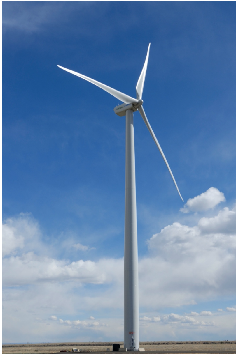
Figure 5. DOE-owned 1.5-MW wind turbine located at site 4.0 at the FC. Photo credit: Jeroen van Dam, NREL
