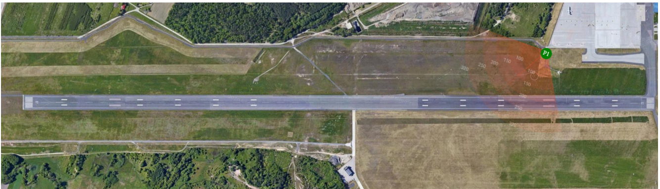
Figure 12. The installation spot depicted as P1 at the airport.
