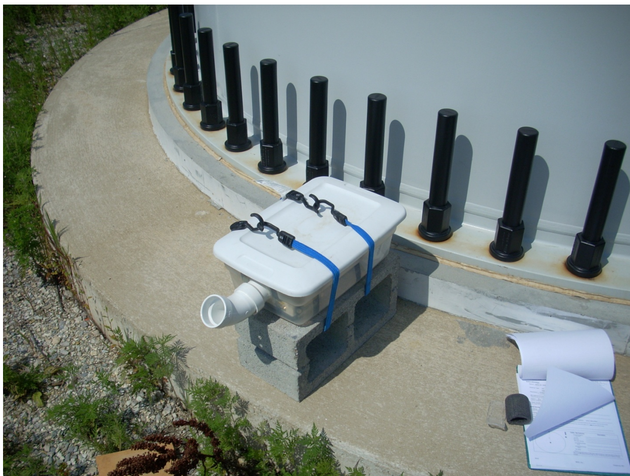
Figure 7. Anabat unit placed at the base of a turbine at the Fowler Ridge Wind Farm.
