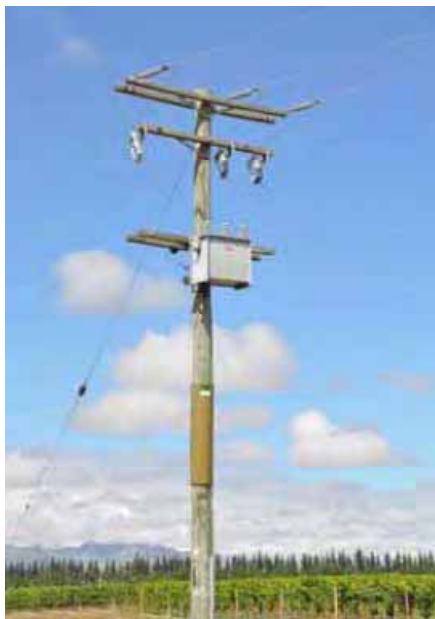
Figure 13: Power pole and transformer box designs known to have electrocuted falcons in the Marlborough region: note the transformer in the picture on the right has been retrofitted with a mitigation device to prevent further electrocutions (Fox & Wynn 2010).
