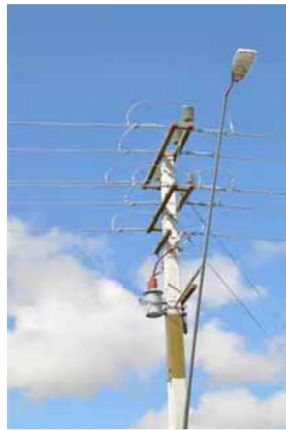
Figure 13: Power pole and transformer box designs known to have electrocuted falcons in the Marlborough region: note the transformer in the picture on the right has been retrofitted with a mitigation device to prevent further electrocutions (Fox & Wynn 2010).
