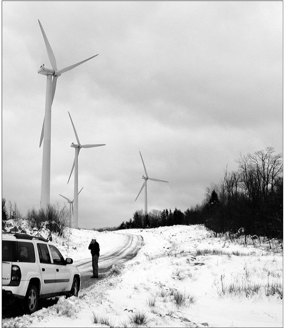
Figure 7: Wind Power Facility in Tucker County, West Virginia
