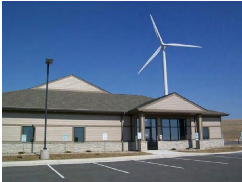
Photo 15. Operations building at the Cedar Ridge Wind Farm. Carcasses were stored in a freezer in the warehouse.
