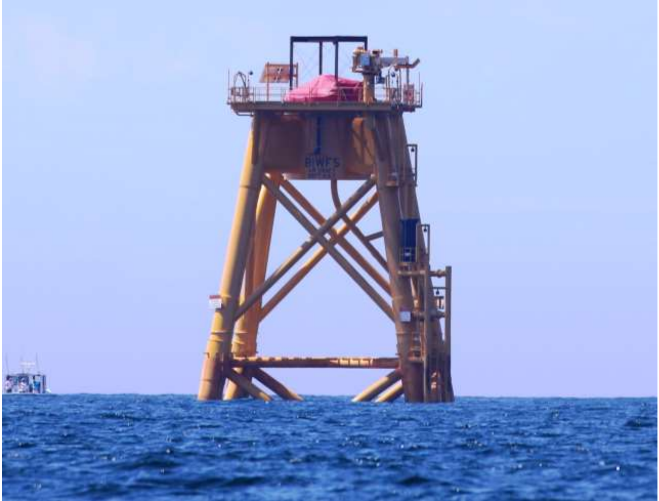
Figure 4. Completed foundation for WTG 5.
