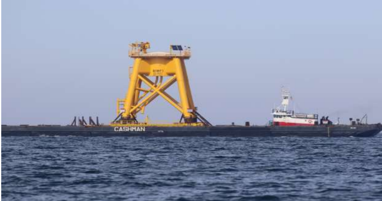
Figure B-9. 09/17/2015 Offshore Photo 2359: WTG 1 steel jacket arriving onsite after being repaired from being struck by a derrick barge after initial installation.
