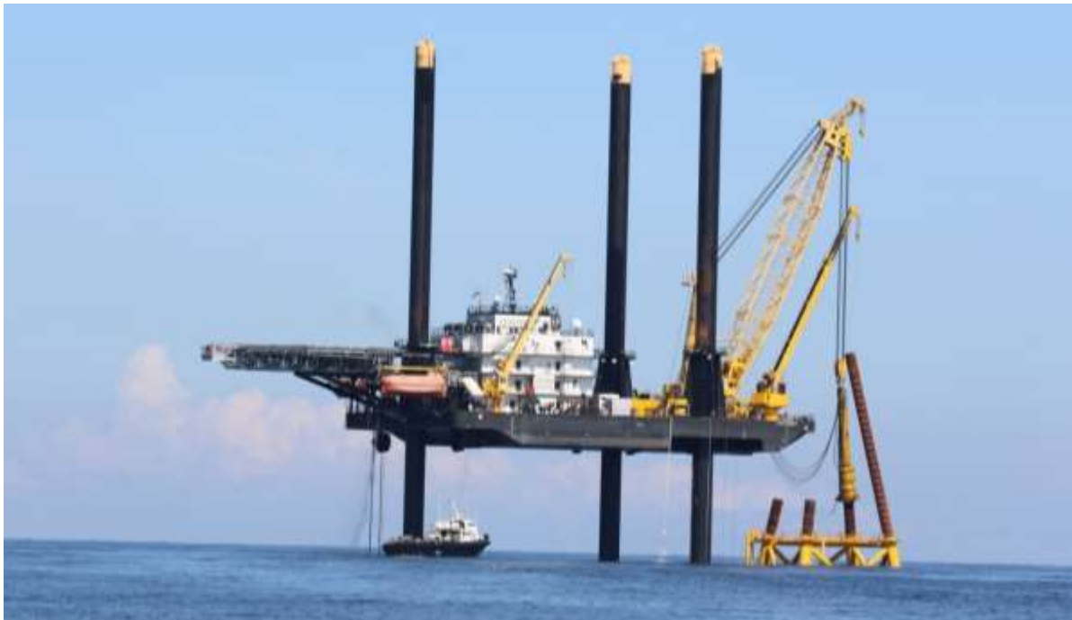
Figure 17. L/B Roberts hammering piles at WTG 1.
