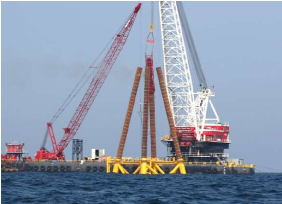
Figure 15. Pileco diesel hammer attempting to drive piles at WTG 2.
