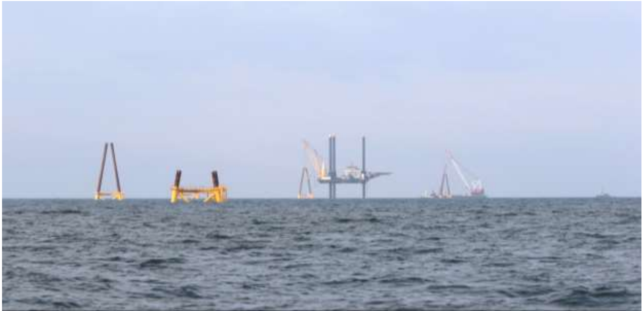
Figure 19. Support vessels at WTG 2 to WTG 5.
