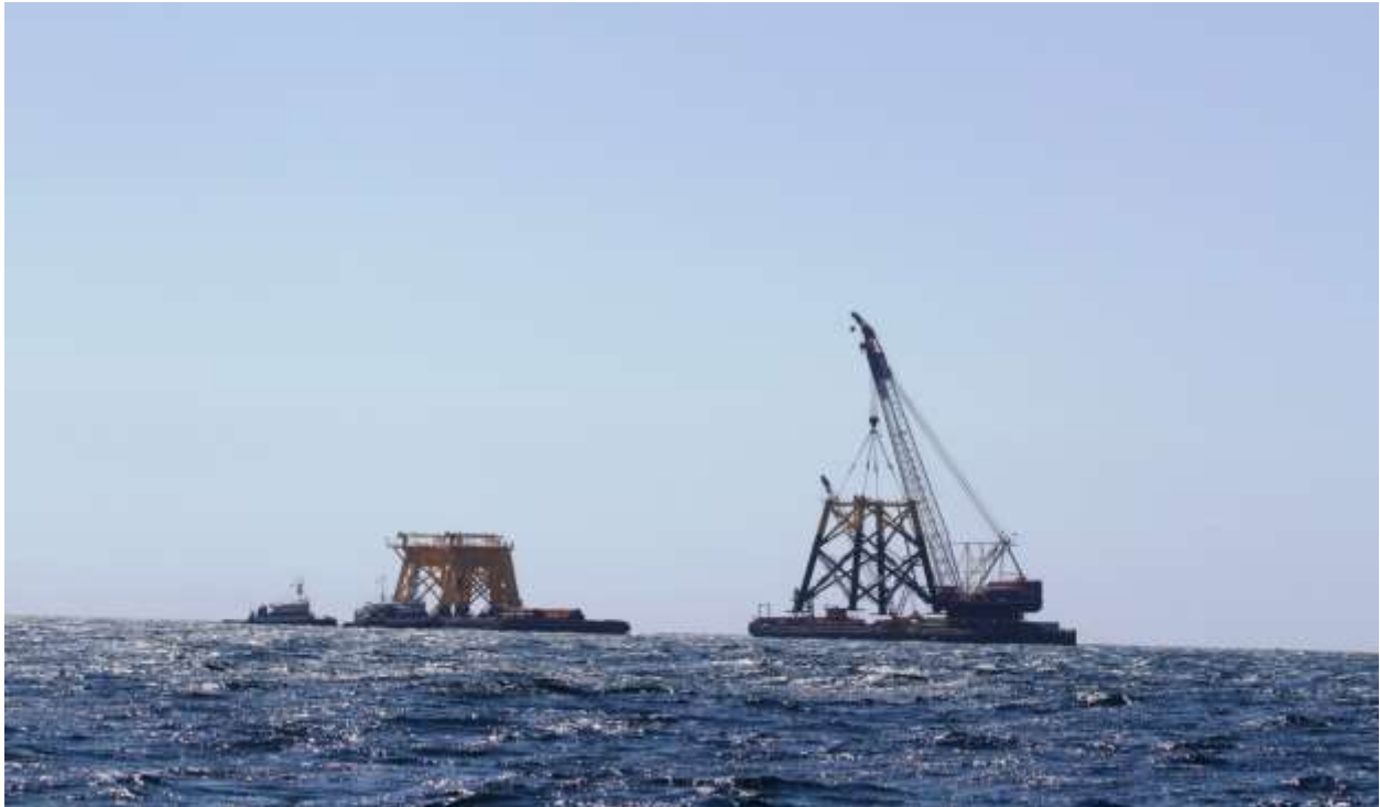
Figure B-2. 9/07/2015 Offshore Photo 3933. Placing WTG 5 steel jacket in the water.
