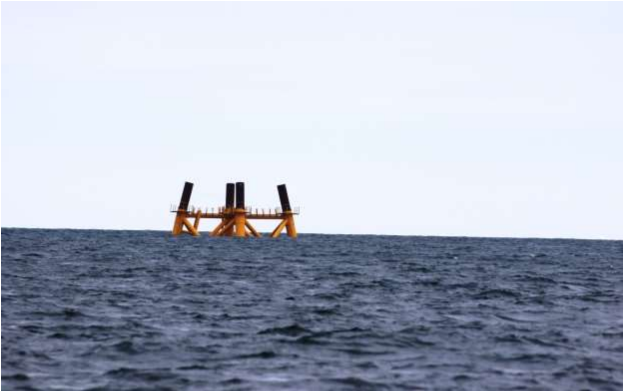
Figure B-22.9/20/2015 Offshore Photo 2584 WTG 1 ready for transition deck.
