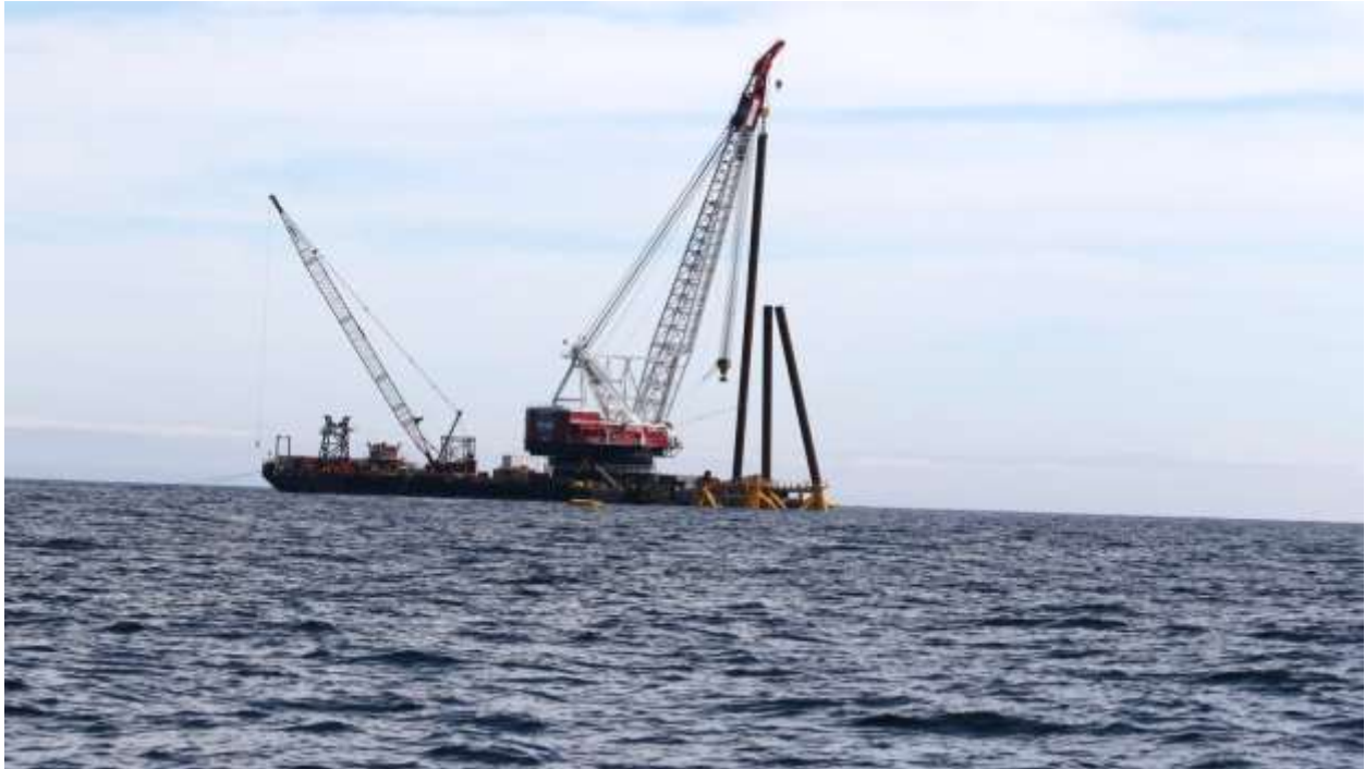
Figure 13. Placing of piles into the WTG 3 steel jacket guide holes.
