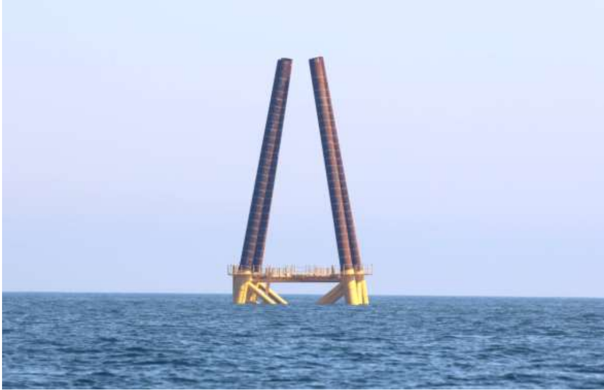
Figure 14. Piles inserted into jacket prior to pile driving.
