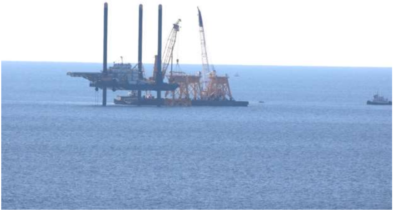
Figure 18. Transition deck installation.
