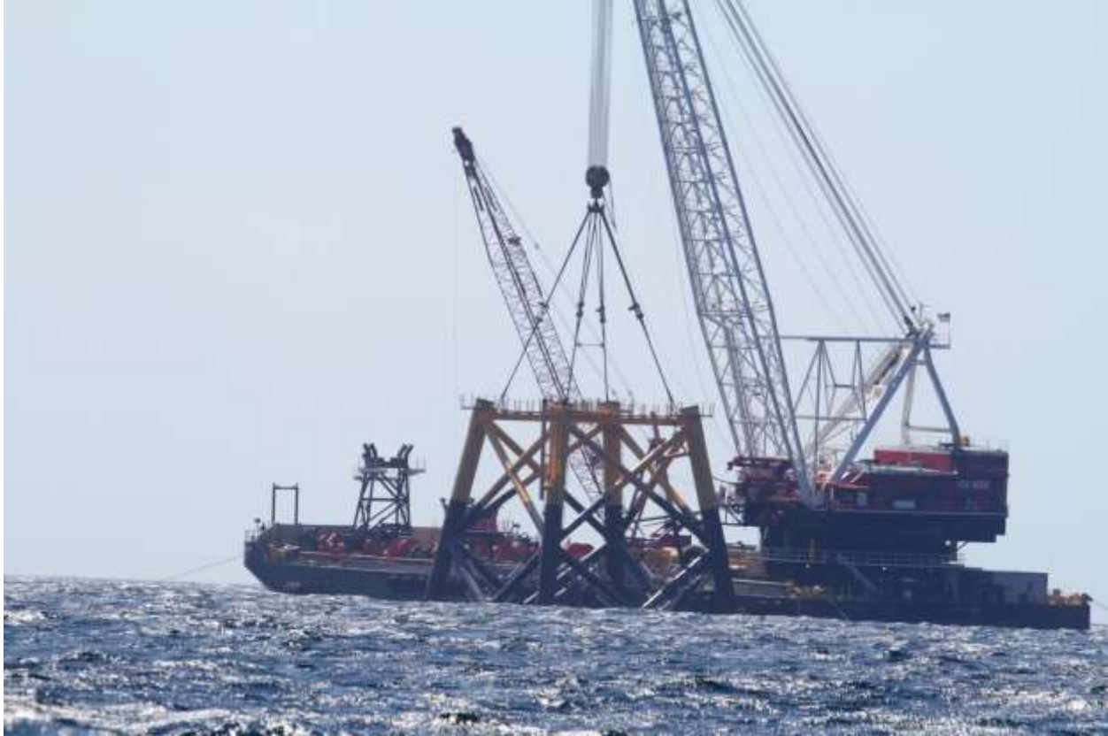
Figure B-3. 9/07/2015 Offshore Photo 3943. Placing WTG 5 steel jacket in the water.
