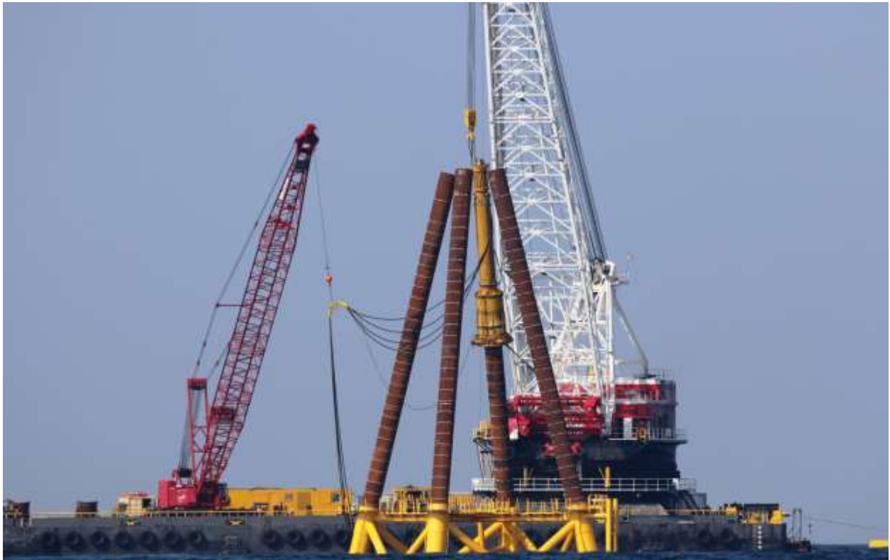
Figure B-14.8/30/2015 Offshore Photo 0692: Pile driving at WTG 3 with hydraulic hammer.
