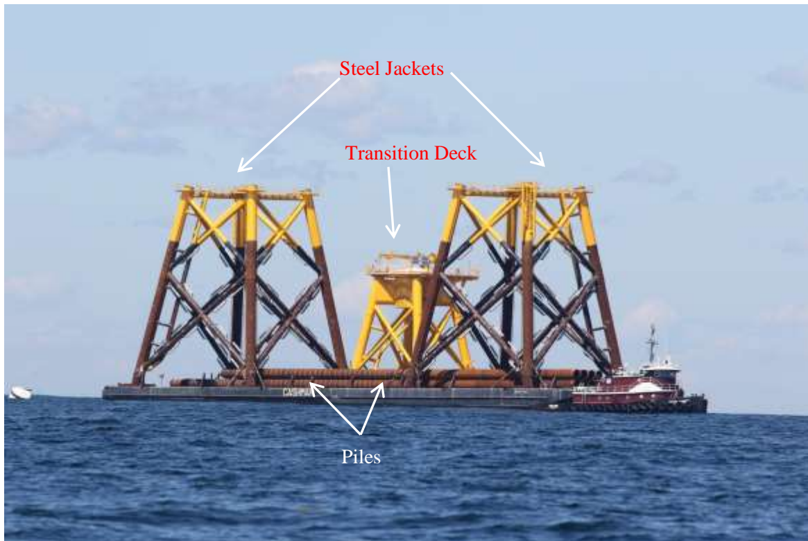
Figure 2. WTG foundations en route to Block Island Work Area.
