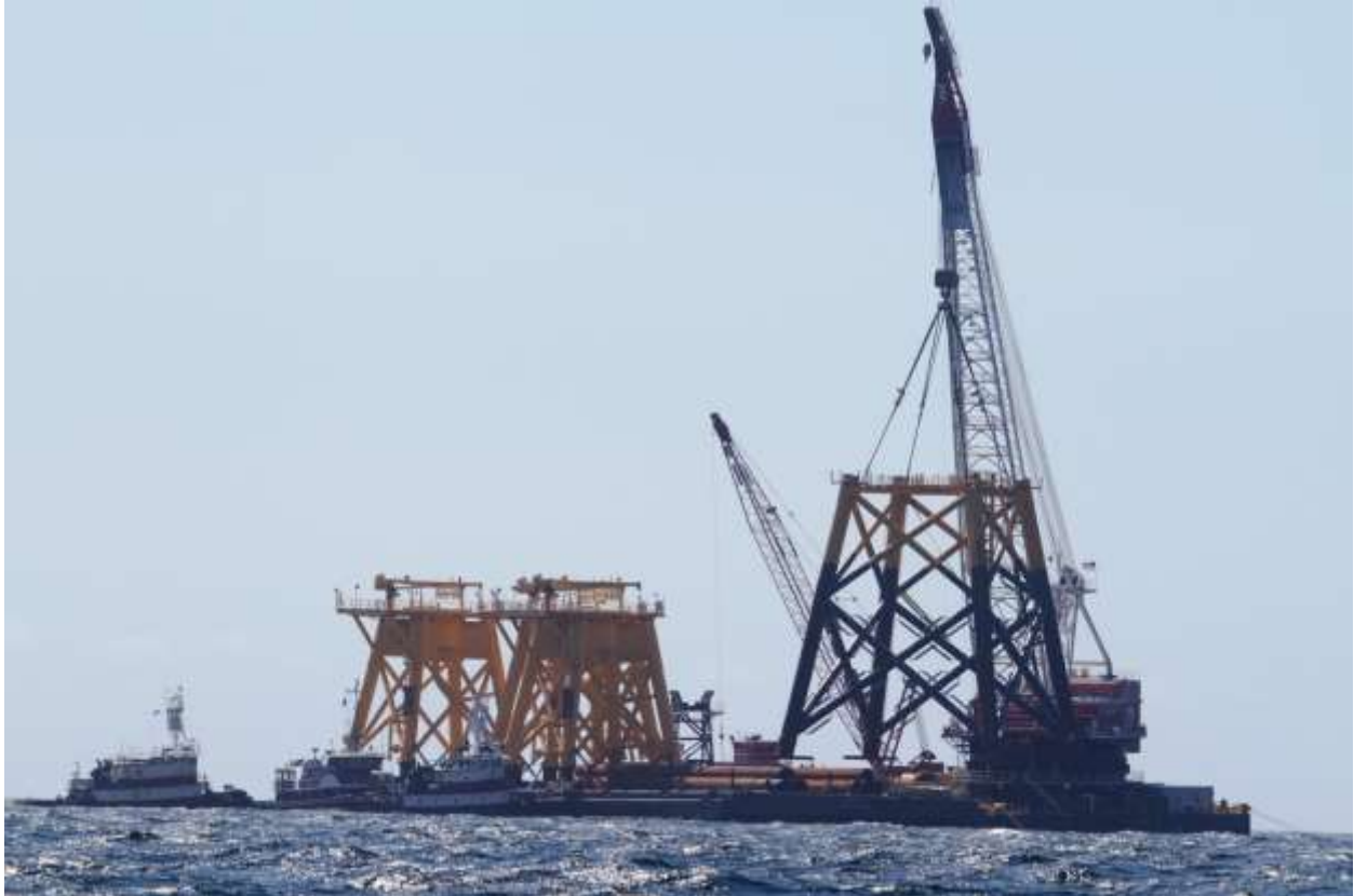
Figure B-1. 9/07/2015 Offshore Photo 3929. Placing WTG 5 steel jacket in the water.
