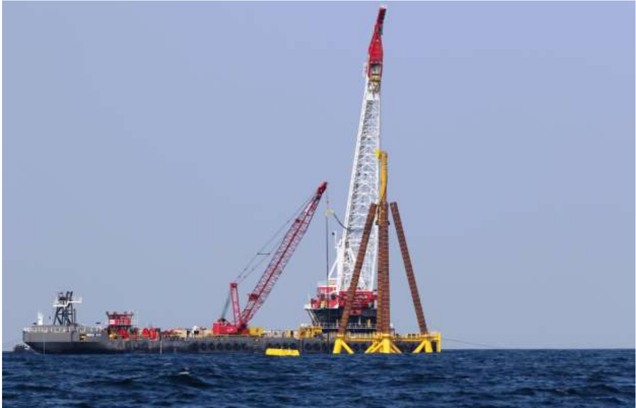
Figure B-13.8/30/2015 Offshore Photo 0679: Pile driving at WTG 3 with hydraulic hammer.
