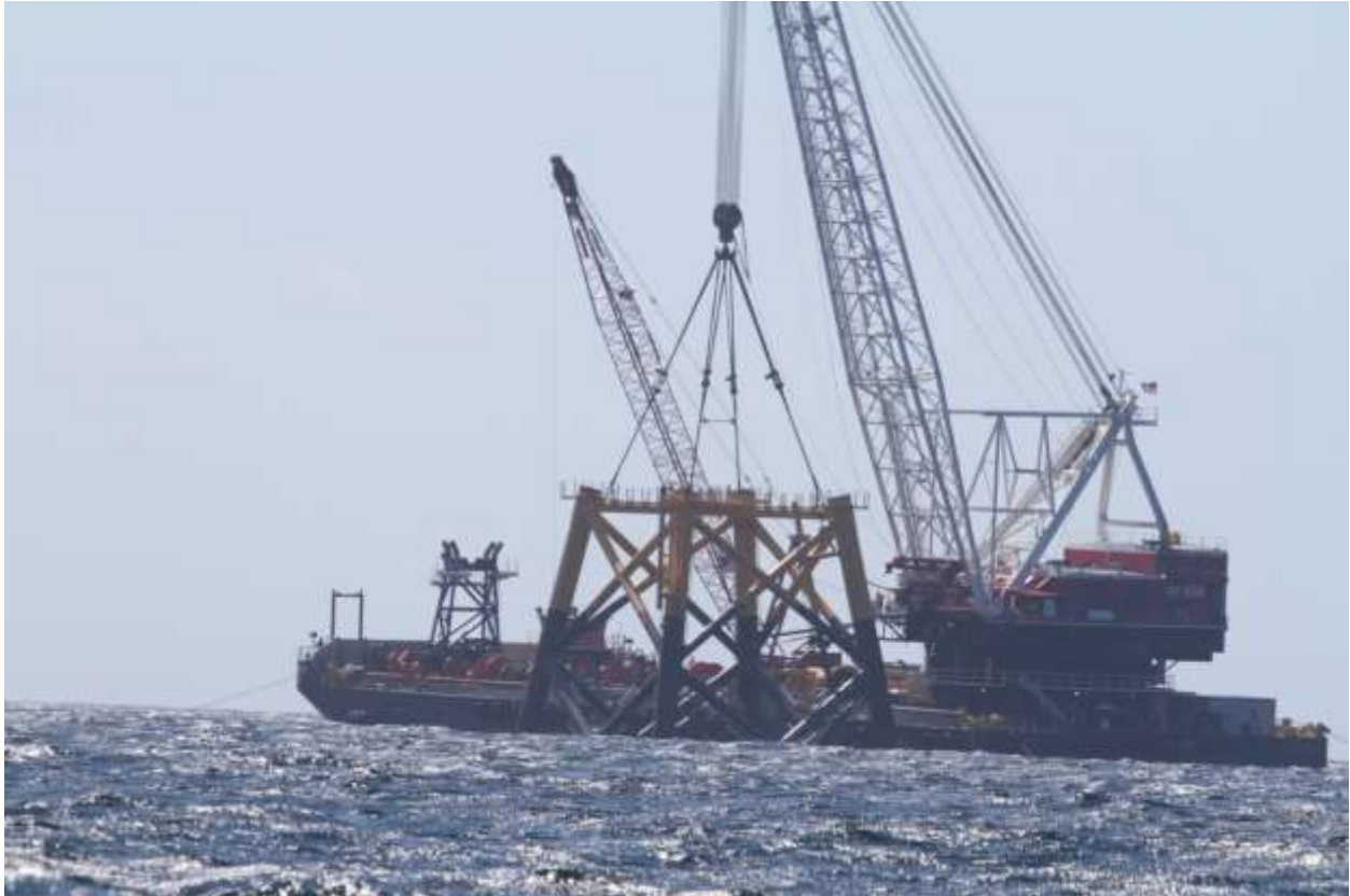
Figure 12. Lowering of the WTG 1 steel jacket into the sea.
