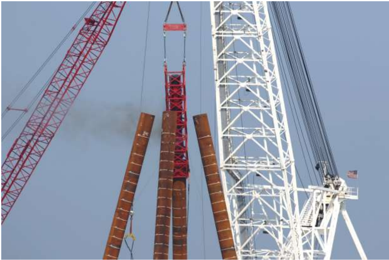
Figure B-6. 08/18/2015 Offshore Photo 0118: Diesel hammer piling at WTG 2.
