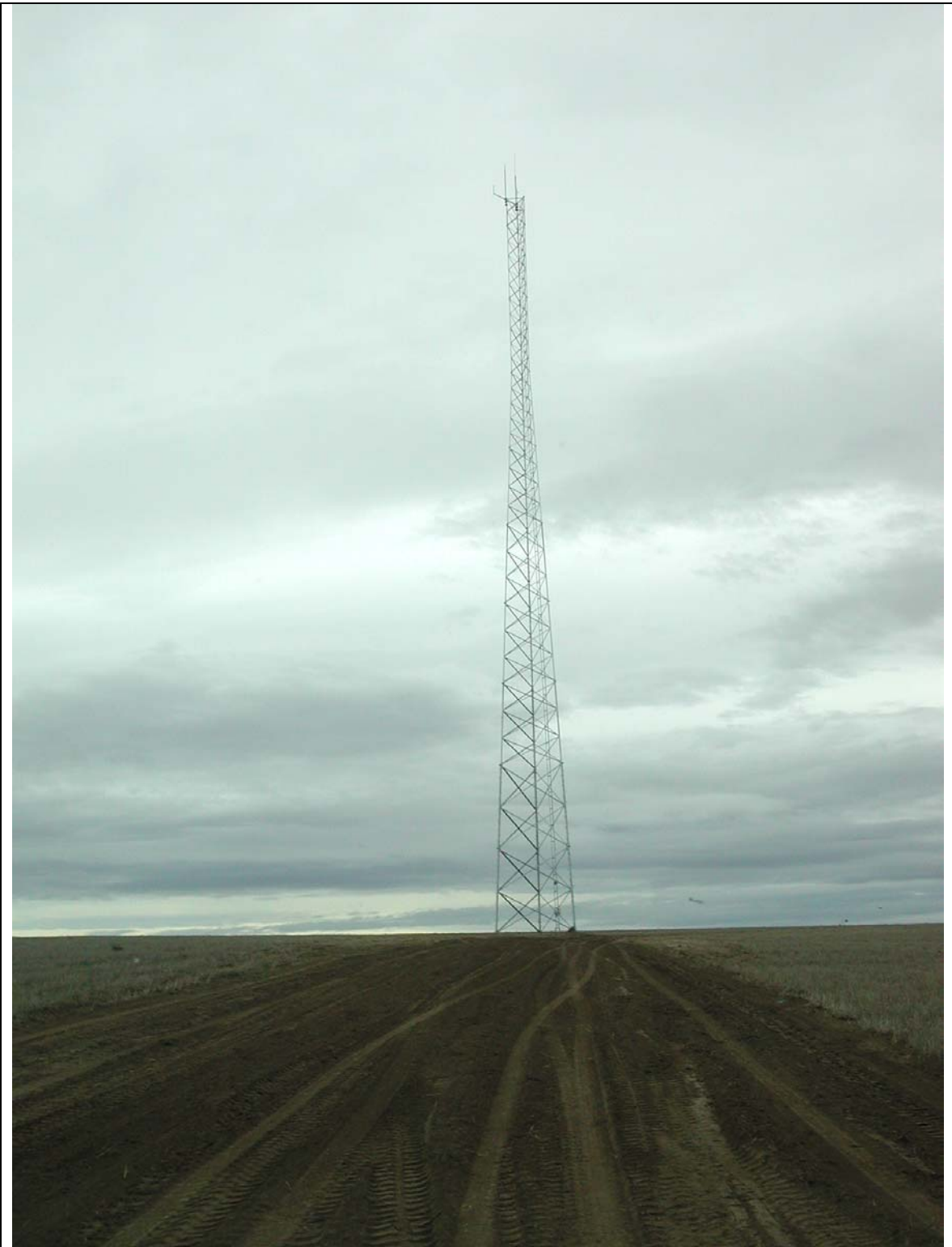
Figure 4. Lattice unguyed meteorological tower at the Nine Canyon Wind Project.
