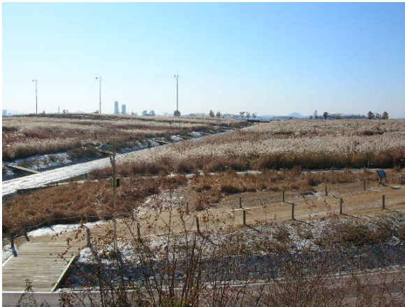
Restored landfill with wind turbines in rear vista, World Cup Park
