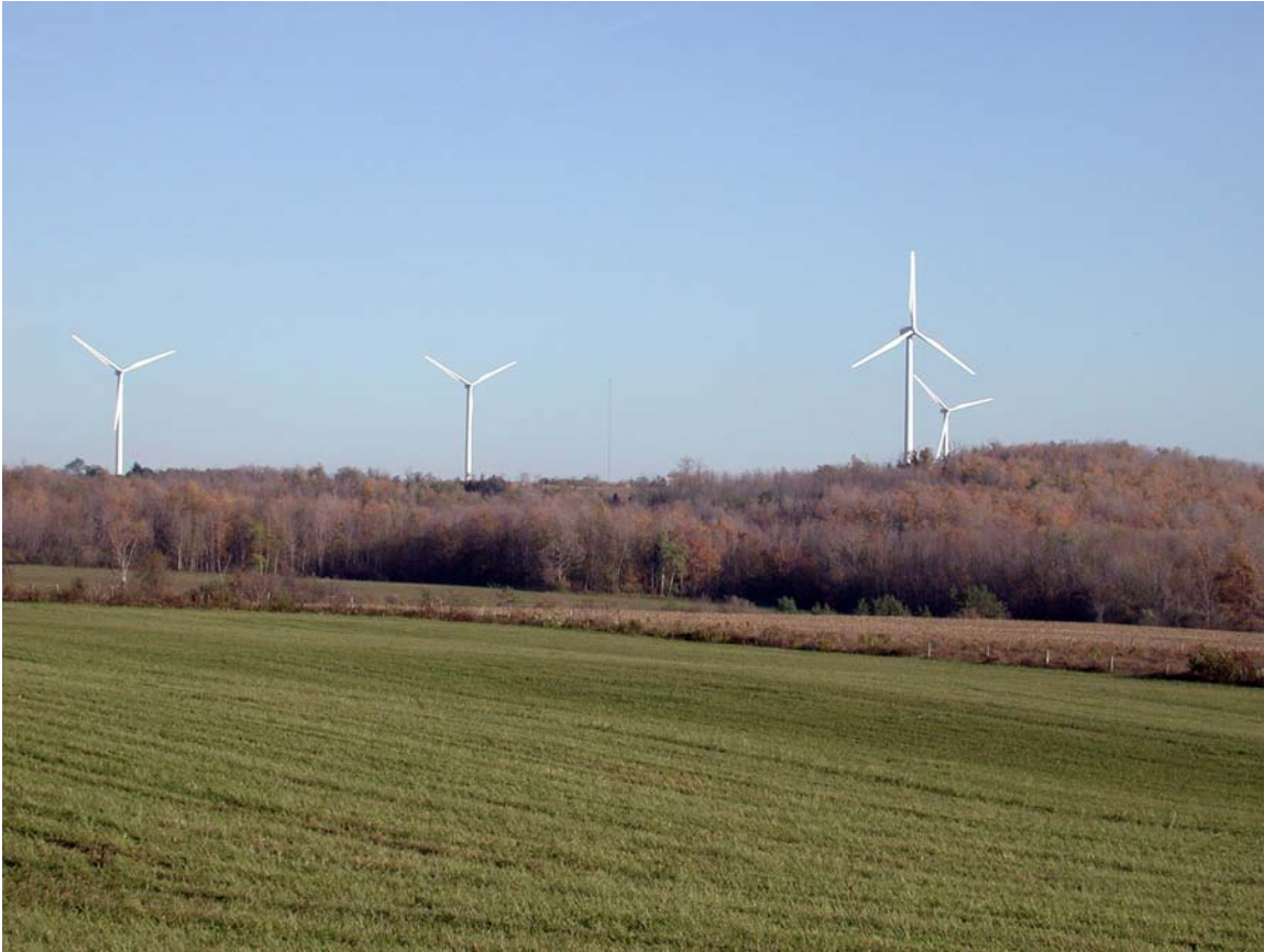
FIGURE D-10 This project in Fenner, NY generally works well in this high-elevation rolling agricultural landscape. The vertical relationship of turbines to distinct hills or ridgelines needs to be examined in simulations. The ridge above does not appear as prominent from most vantage points, but the issue could arise in other situations. Source: Photographs by Jean Vissering, Jean Vissering Landscape Architecture.
