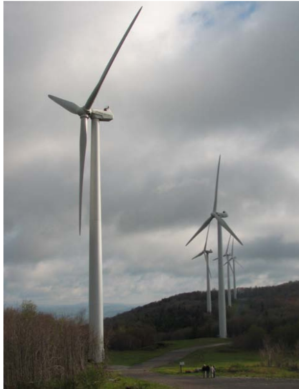
FIGURE 3-3 Mountaineer Wind Energy Center, WV. The 5 turbines in this photograph are at the southwest end of the array of 1.5 MW turbines; they are at the lower left of the aerial view in Figure 3-7. Photograph by David Policansky.
