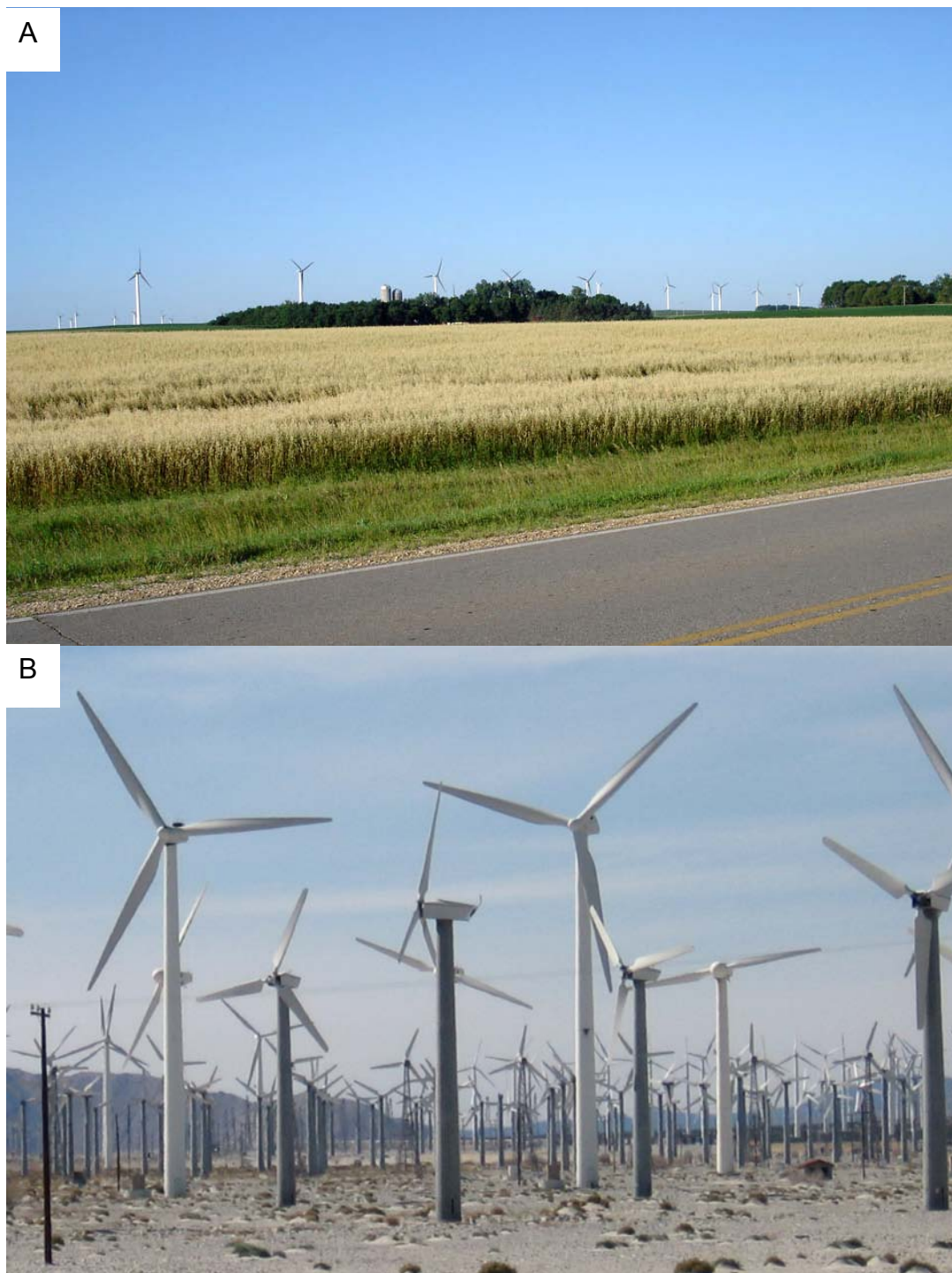
FIGURE D-12 (A) The repetition of identical elements that is characteristic of wind energy projects helps to create a sense of order. (B) The valley location at San Geronio (Palm Springs, CA) diminishes the scale of this large project, but the overall accumulation of different turbine types results in a much more cluttered appearance than is likely in future project planning and maintenance. Sources: (A) Photograph by Sandy Wobeck, East Montpelier Gully Jumper; (B) Photograph by David Policansky.
