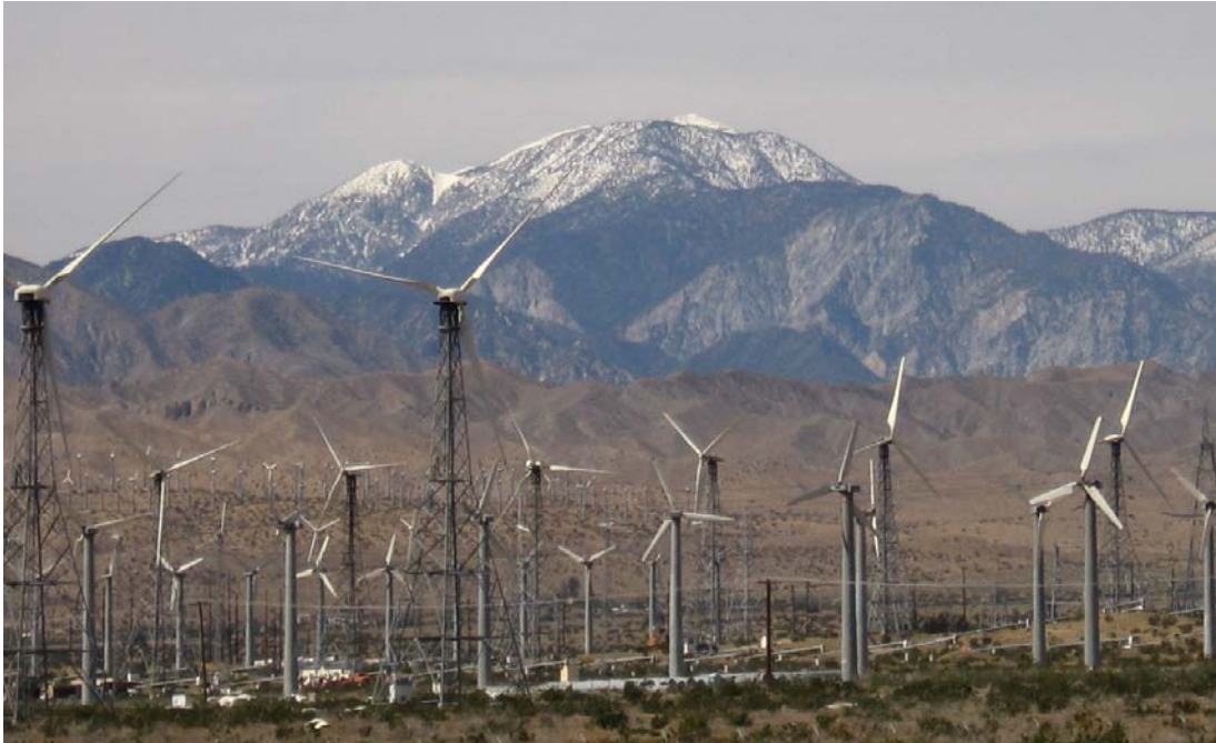
FIGURE 3-2a Turbines at San Geronio showing lattice and monopole towers. Photograph by David Policansky.
