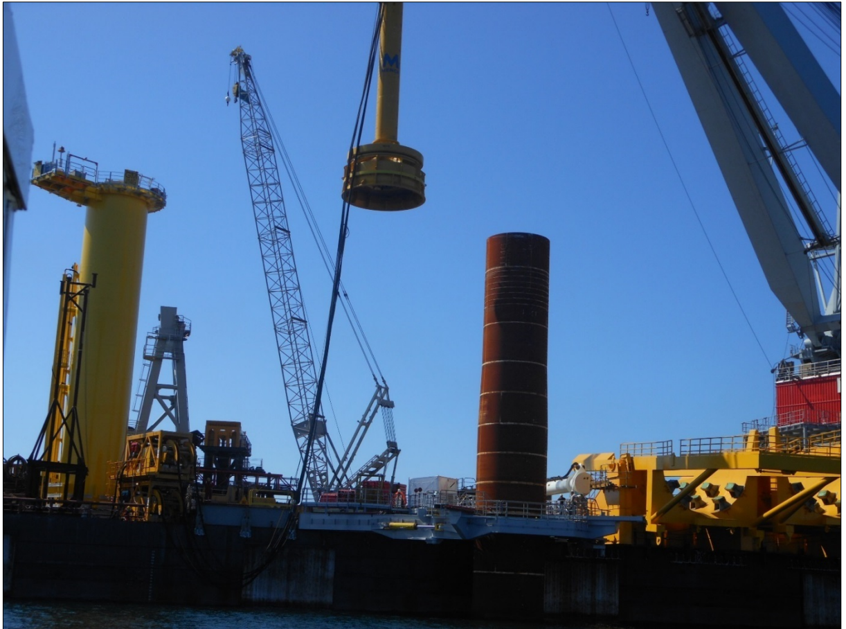
Figure 4.1: Hammer piling of a monopile
