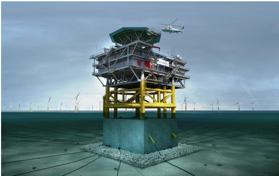
Figure 11: Hybrid foundation.
