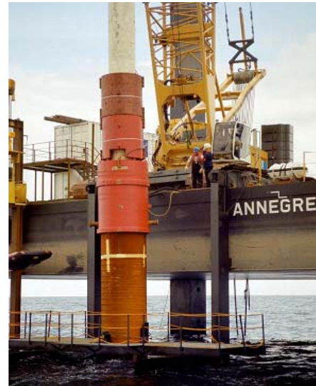
Fig. 1: Hydraulic hammer on a pile of FINO1.
