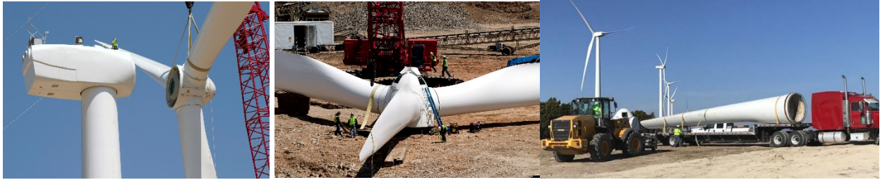
Figure 4-1 Wind turbine blade decommissioning
