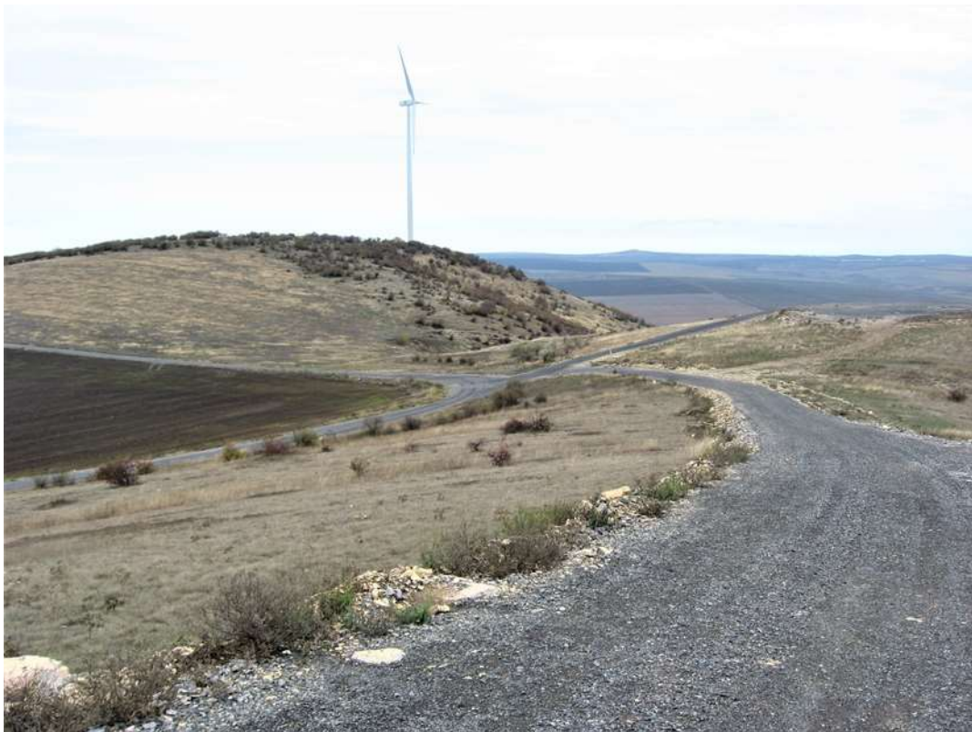
Figure 5-1 Habitat loss and fragmentation by construction platforms and access roads in hilly steppe landscape
