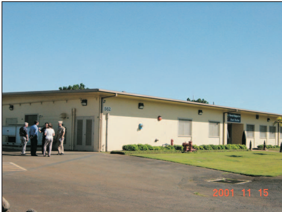
Building 562. Equipment shelter located inside double doors to the right of the group of people visible in the photograph.
