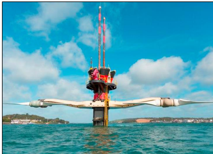
Figure 2.1. SeaGen Tidal Turbine installed in Strangford Lough, Northern Ireland. The first commercial scale grid connected tidal turbine in the world. In the image the two twin-bladed rotors (white parts) have been raised above the water so they can be accessed from the pile (red part). During operation the two rotors are lowered into the water and turn to produce energy from the passing tide.
