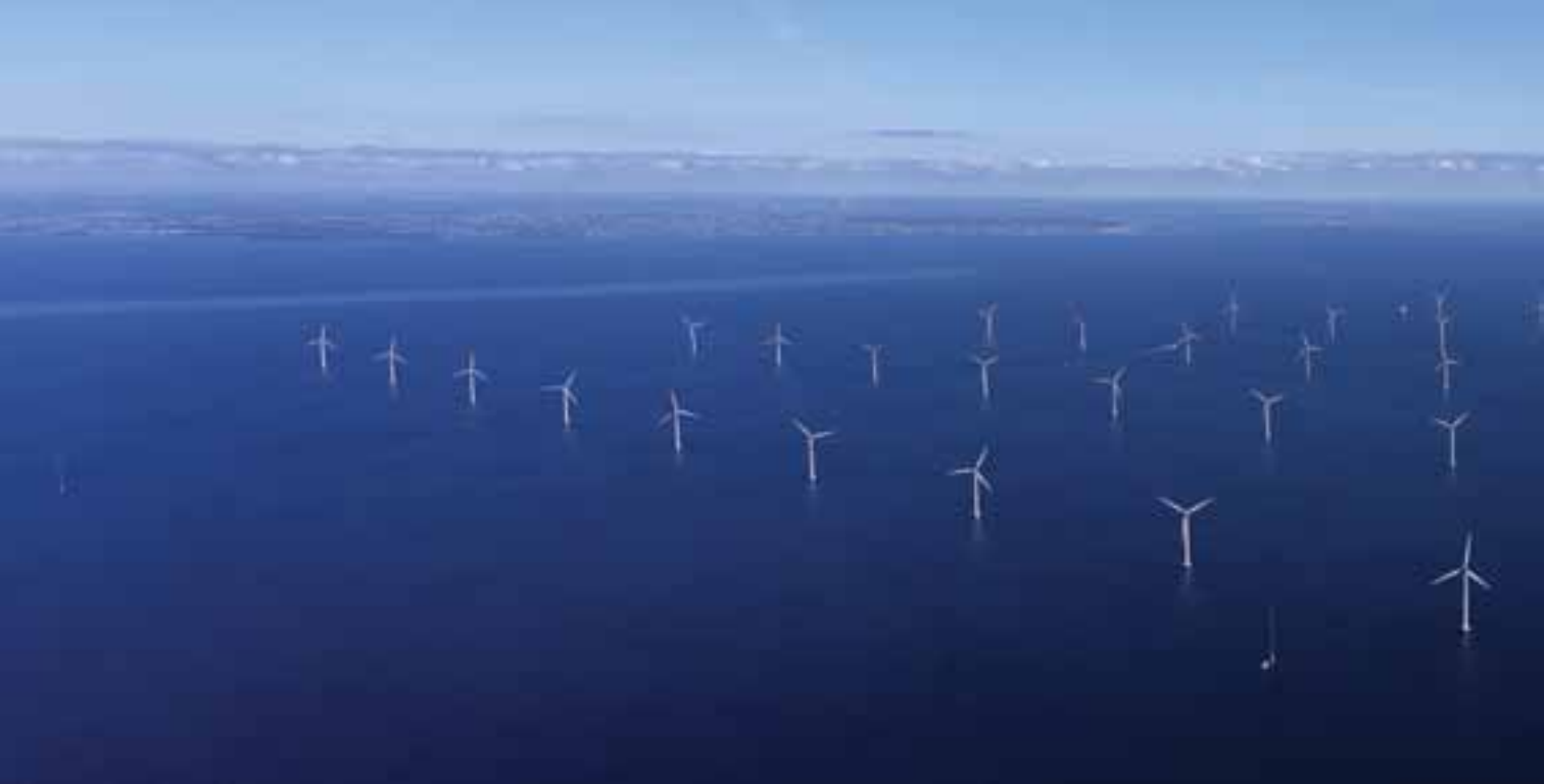
FIGURE 1.10 Nysted Offshore Wind Farm. PHOTO: NYSTED OFFSHORE WIND FARM
