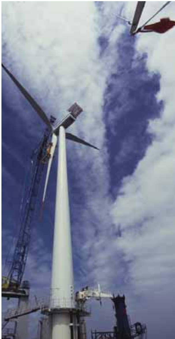
FIGURE 1.4 Construction of wind turbine at Horns Rev.
