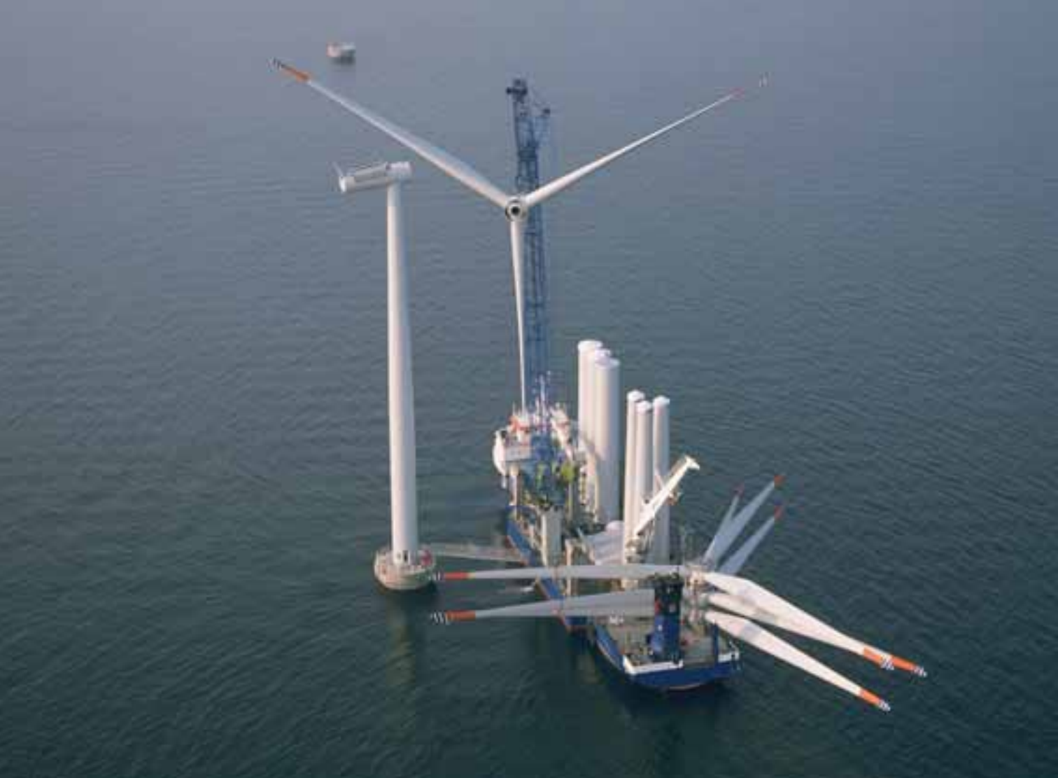
FIGURE 3.9 Construction of the first wind turbine at Nysted Offshore Wind Farm
