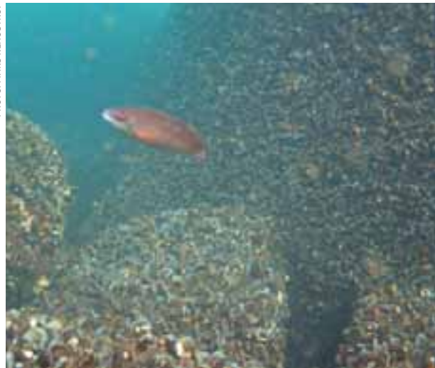
FIGURE 1.5 Scour protection with common mussels at Nysted.
