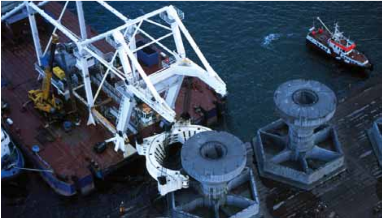
FIGURE 3.7 Photos of the turbine foundations before they were positioned on the seabed.
