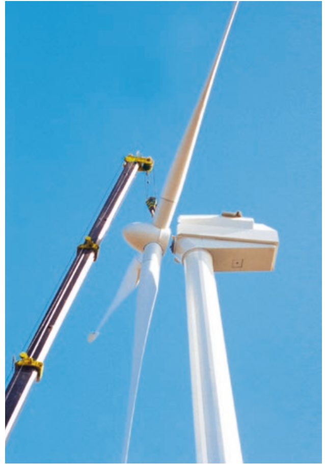
Figure 10. Turbine Construction. (Source: SEAI)
