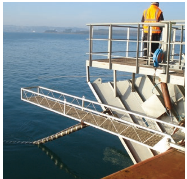
Figure 11. Laying Cable at Sea. (Source: SEAI)
