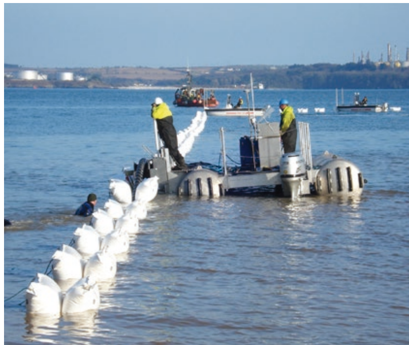
Figure 4. Floating a Cable to Shore. (Source: SEAI)
