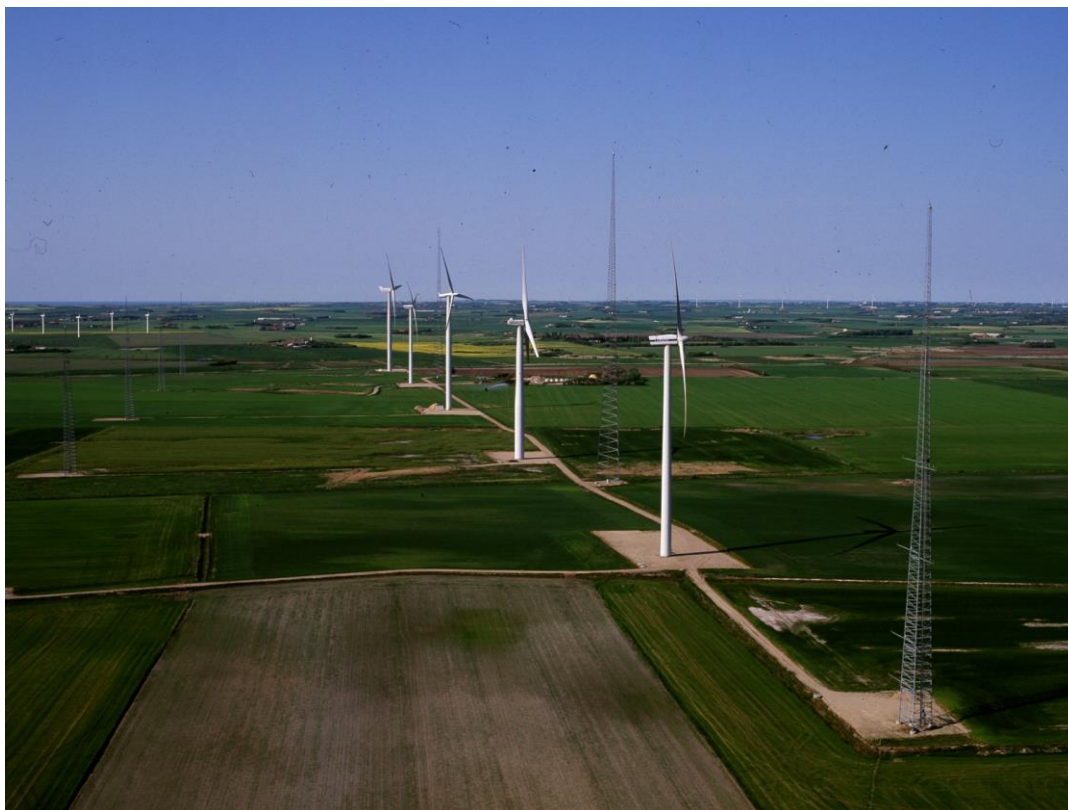
Figure 24 The row of wind turbines at the Høvsøre test site with the tall met. mast in the front.
