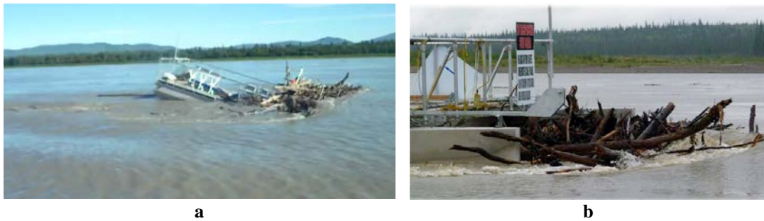
Figure 5. Debris accumulation on the bow of the 5 kW New Energy EnCurrent turbine barge at Ruby, Alaska (Pelunis-Messier 2010) (a); debris accumulation in front of a 25 kW New Energy turbine barge at Eagle, Alaska (photo credit: Alaska Power & Telephone) (b).
