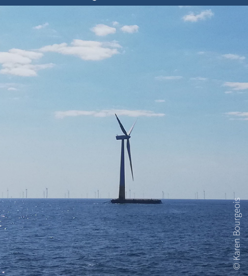
View of the Floatgen floating wind turbine in the foreground and the Saint-Nazaire offshore wind farm in the background
