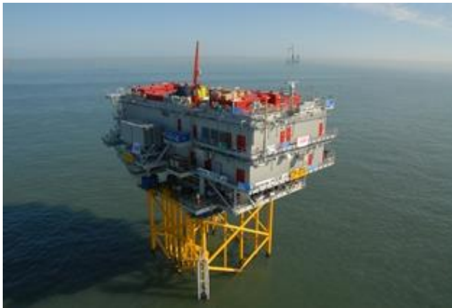
Figure 2: the 4 storey 2000 T offshore transformer station (OTS) was installed on 16 March 2012
