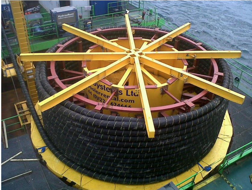
Figure 5: export cable B on the cable laying vessel (3 July 2012)
