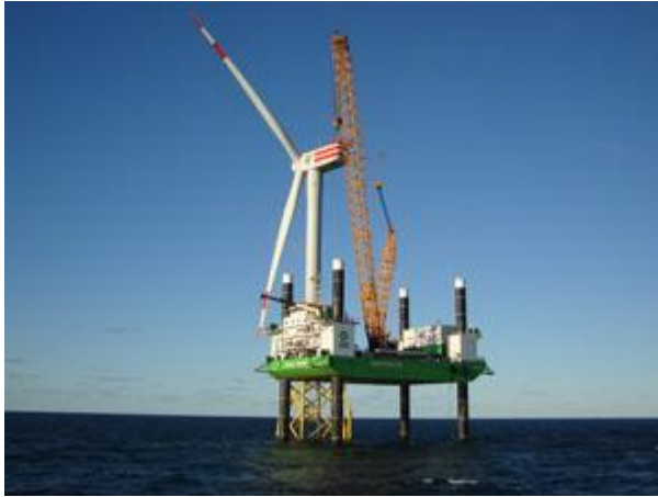
Figure 4: “Neptune” installed the first of 30 WTG (6,15 M) on 21 March 2012
