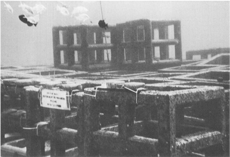
Figure 3. Open framework concrete cube artificial reef comprised of 42 modules. Modules are 1.2 m on a side and weigh 1,150 kg.
