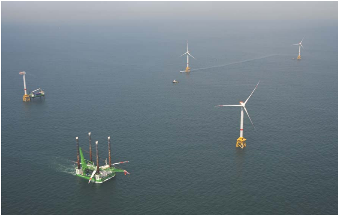
Turbine transport and installation on the Thorntonbank
