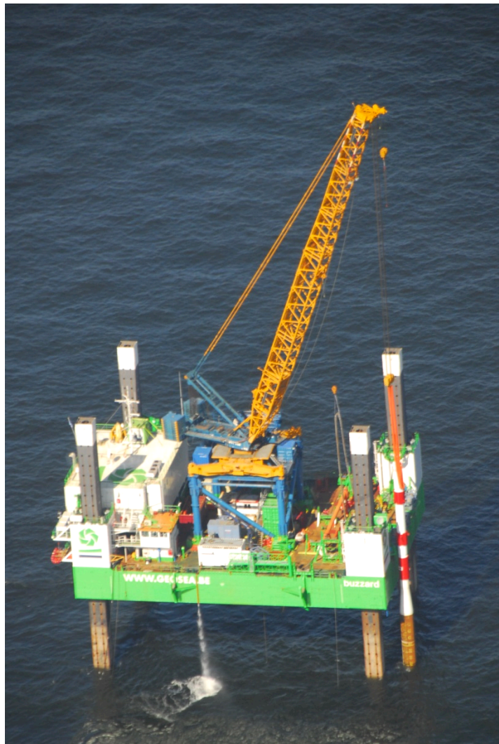
Piling of a pinpile on the Thorntonbank
