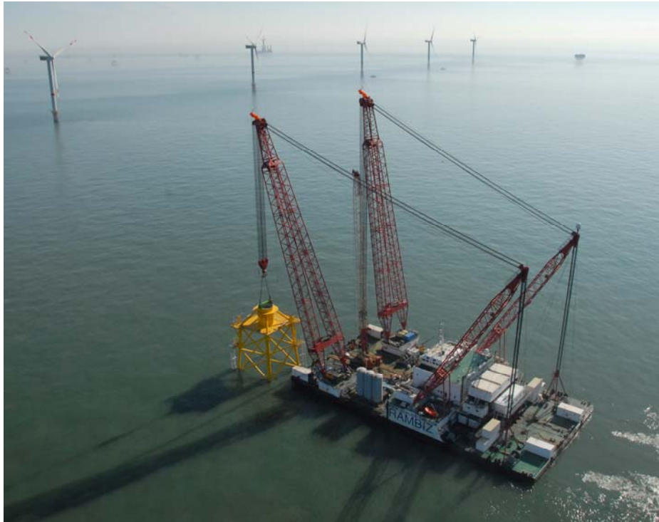
Figure 3. Phase III jacket installation (Photo C-Power).
