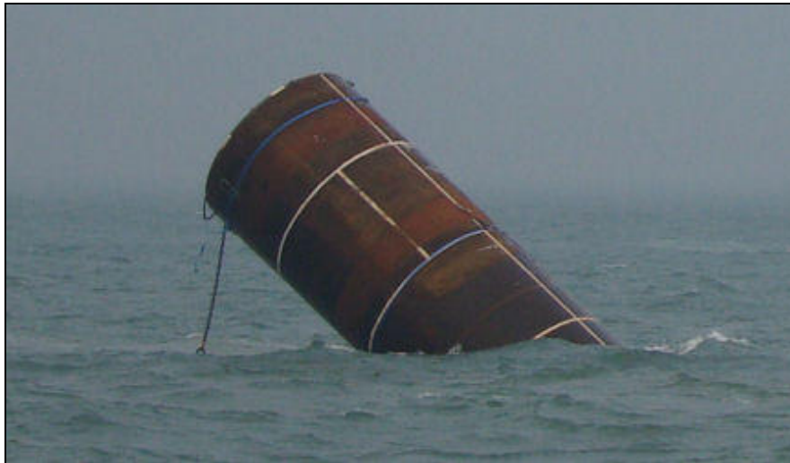
Figure 9. Two monopiles sank during the transport from the port of Zeebrugge to the Blich Bank. MP C05, which was lost on October 24 th , remained partially above the water surface (Photo Belwind).
