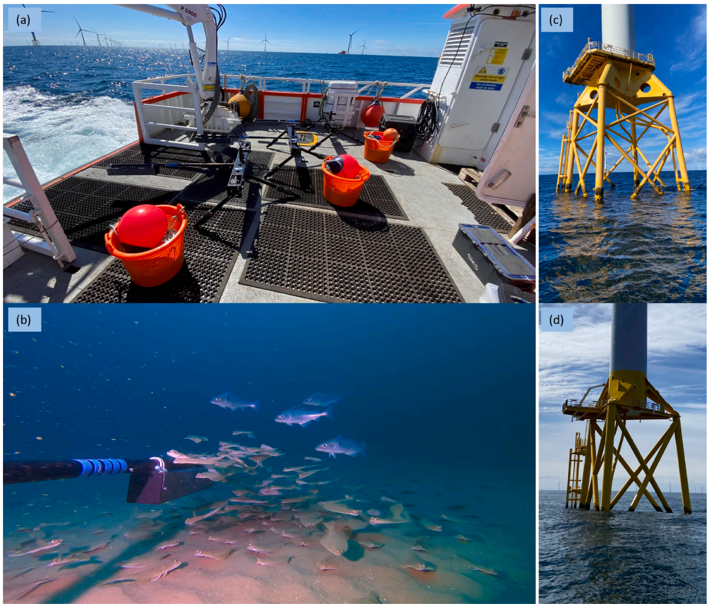
Fig. 2. (a) Baited remote underwater video systems used for the offshore wind farm surveys. (b) Example image from BRUV video footage illustrating main species composition and abundance (haddock and flatfish). (c) Four leg turbine jacket at Beatrice wind farm, and (d) three leg turbine jacket at Moray East wind farm.
