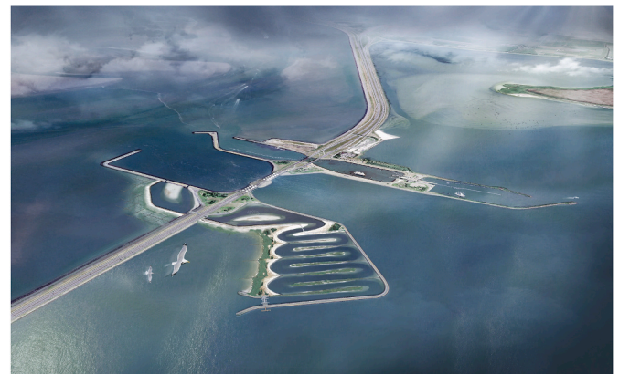
Fig. 4. Conceptual image of the proposed Fish Migration River adjacent to the Kornwerdezeand sluices and navigation lock on the Afsluitdijk, Netherlands (reproduced with permission of Provincie Fryslân, the Netherlands – Feddes/Olthof – Landschapsarchitecten).
