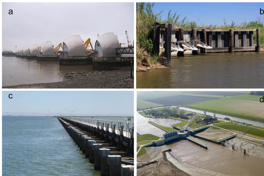
Fig. 2. Examples of tidal barriers including: a) the Thames River surge barrier, England (photograph by T. Corser, distributed under CC-BY/SA 2.0 license United Kingdom. Image cropped); b) tide gates, Louisiana, USA (M. Kimball); c) Tauwitschere Barrage, Australia (C. Bice); and d) Nieuwe Statenzijl, Netherlands (reproduced with permission of RWA Hunze en Aa’s, Netherlands).
