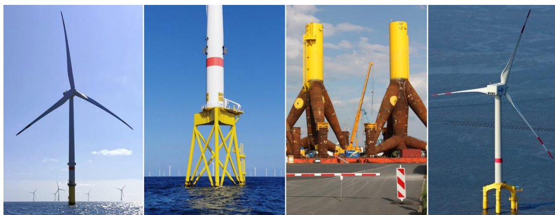
Figure 13: Foundations of OWTGs. From left: Monopile, Jacket, 4-legged Tripod, Tri-pile (photo far right: Martina Nolte, CC BY-SA 3.0 de, all others: itap GmbH).
