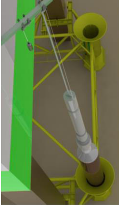
Figure 6.7 - Pile hammer installing a pile
