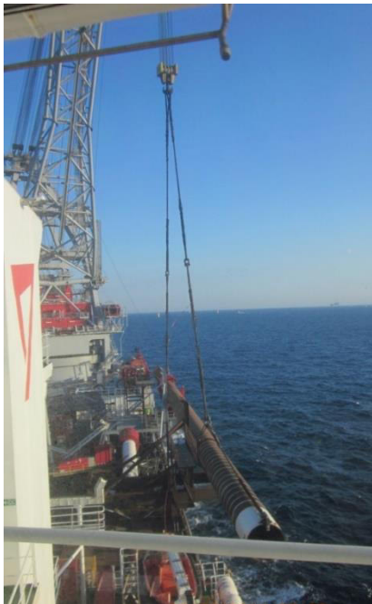
Figure 6.6 - a) Pile being up-ended ready for deployment and b) being deployed into the PIF
