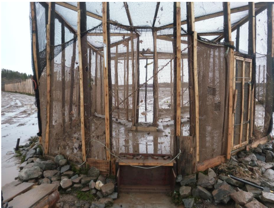
Figure 6: Bramber weir trap net and gate used to drain water and collect fish.
