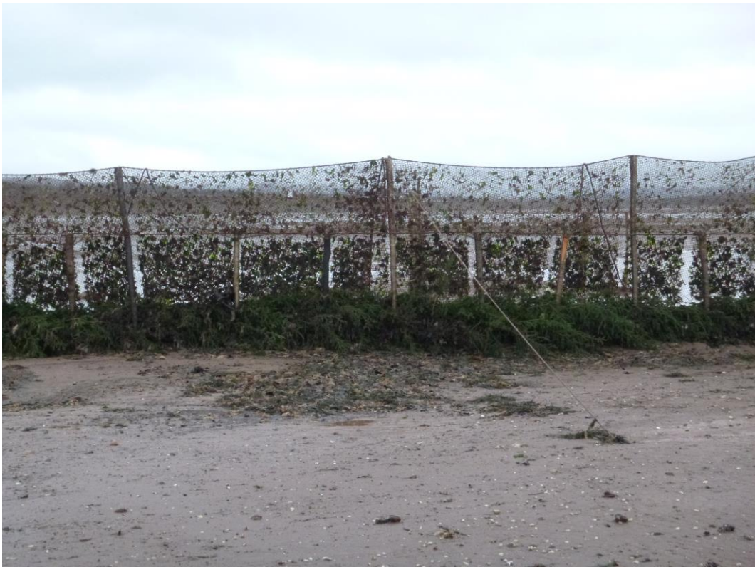
Figure 4: Photo showing the structural composition of the Five Islands weir.
