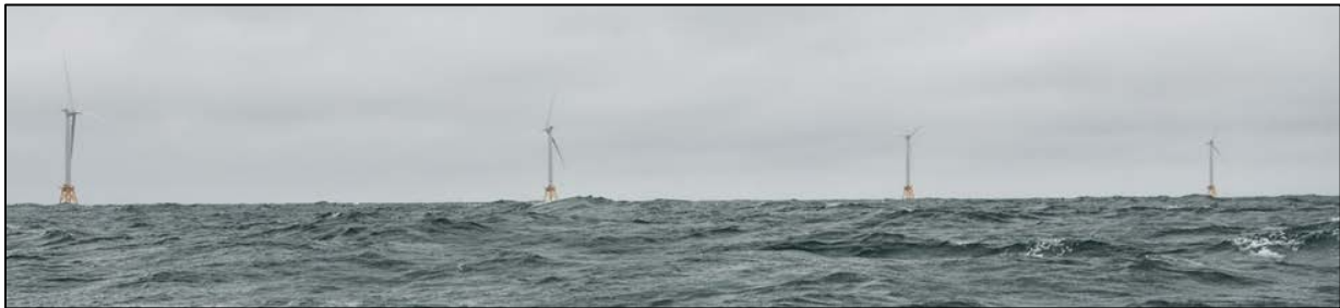
Figure 25. Block Island Wind Farm with jacket substructures, showing 0.5 mi (0.8 km) turbine spacing.
