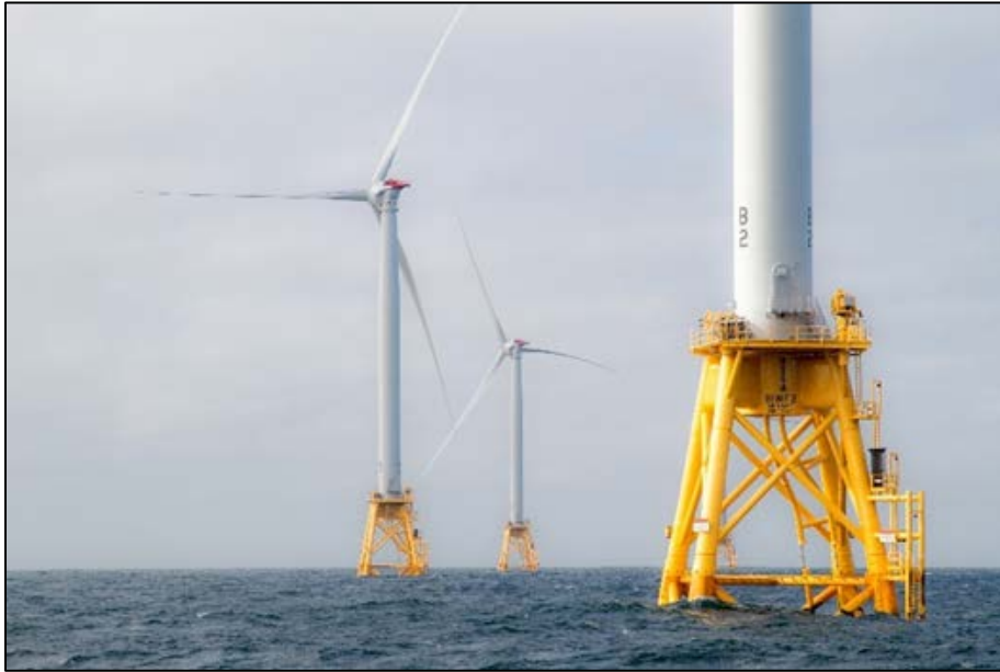
Figure 40. Fixed-bottom jacket substructures that were manufactured in the Gulf of Mexico region for the Block Island Wind Farm.
