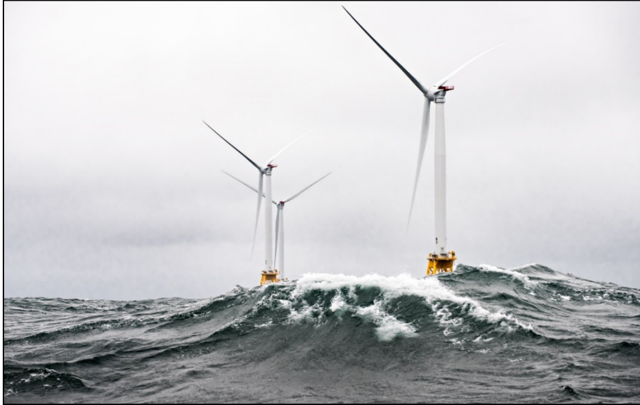
Figure 26. Block Island Wind Farm with jacket-type substructures (yellow). Photo credit: Dennis Schroeder, NREL.
